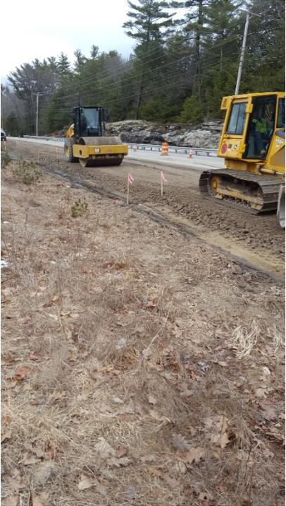
Rough grading and compaction of road base gravel in the left lane, looking east
