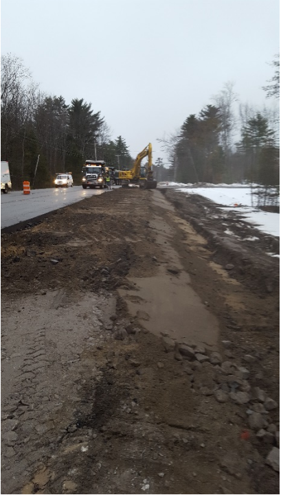
Removing pavement and grubbing top soil in the left lane, looking north
