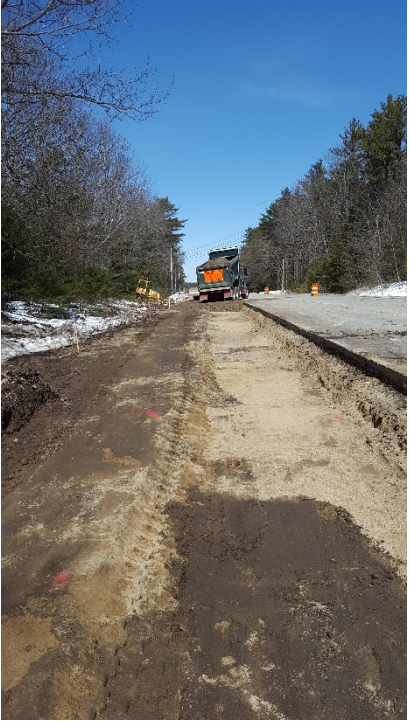
Subgrade graded, gravel step constructed, in the left lane, looking north
