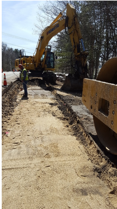
Grading subgrade material in the left lane, looking south
