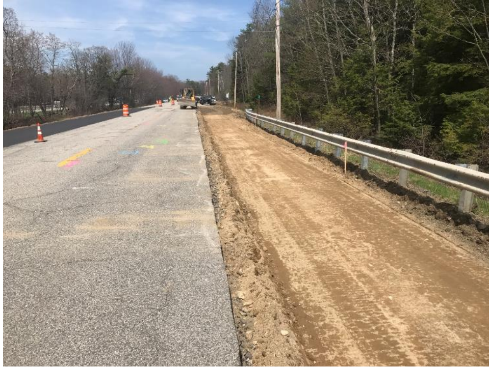
Photo 1 – Looking north, northbound shoulder excavated
