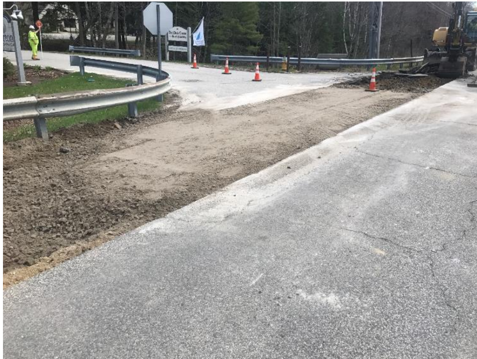
Photo 2 – Half of Norton Insurance driveway made passable to traffic while excavating opposite lane.
