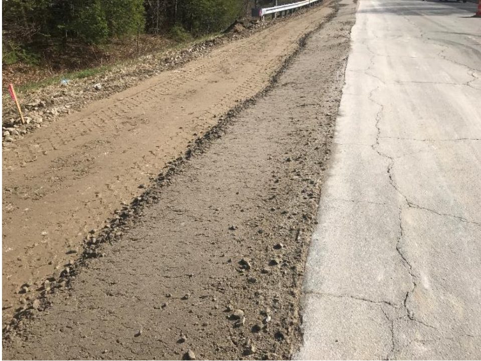
Photo 3 – gravel paced to match roadway.
