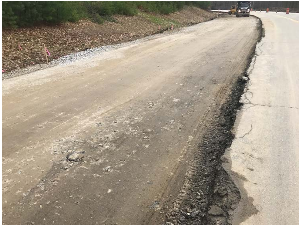
Photo 2 – Near +/- sta. 139+00 looking south, area rough graded and compacted
