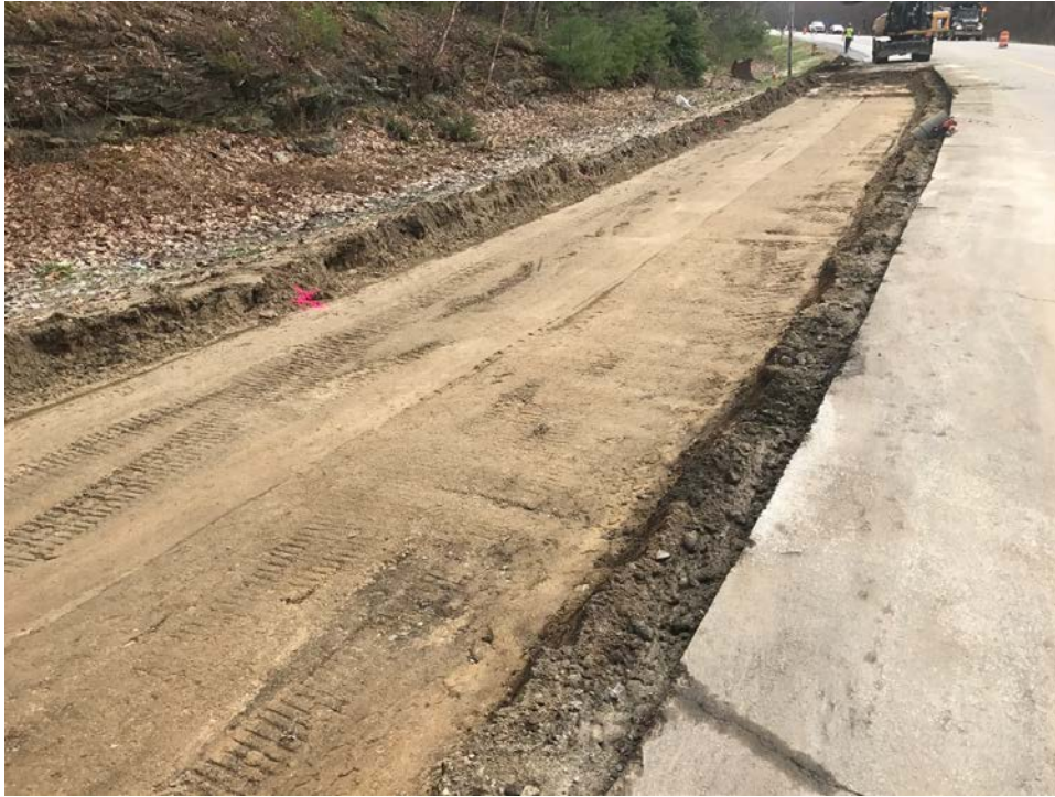
Photo 3 – Near +/- sta. 134+50, shoulder area excavated to subgrade.
