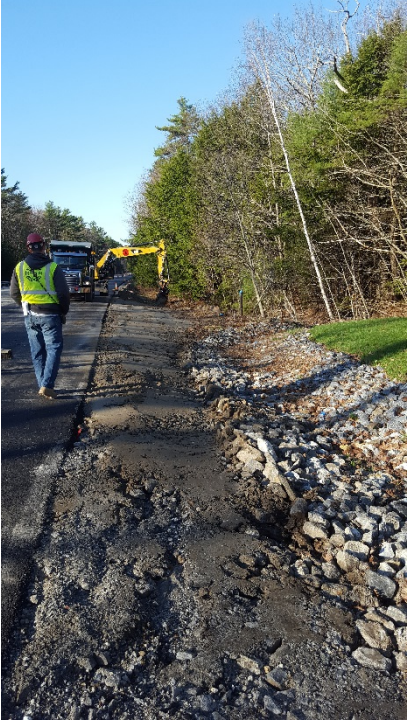
Installing loam on the shoulder slopes in the left lane, looking south
