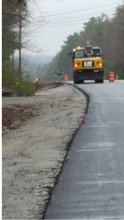
Installing loam on the shoulder slopes in the left lane, looking north
