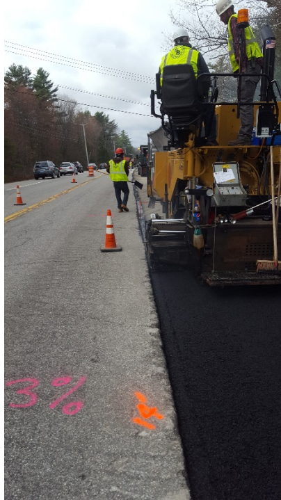
Paving the base lift in the left lane, looking north
