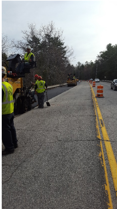
Paving the base lift in the left lane, looking north
