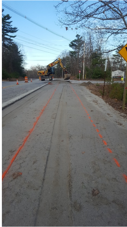
Break of sloped in box cut marked out for paving in the left lane, looking south
