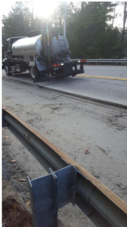
Tack installation on the saw cut joint in the left lane, looking north
