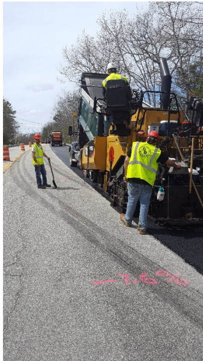
Paving the intermediate lift in the left lane, looking south
