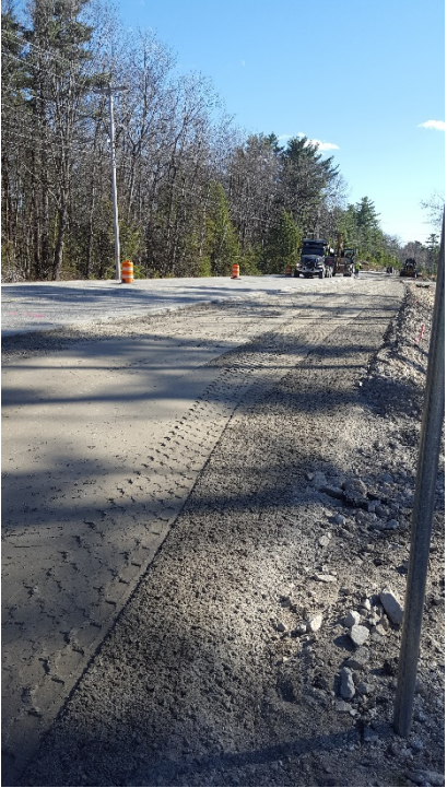
Graded base gravel in the left lane, looking south
