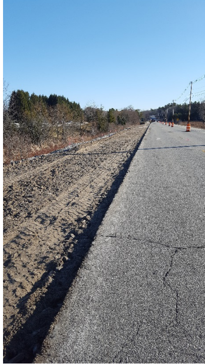
Graded base gravel in the left lane, looking north
