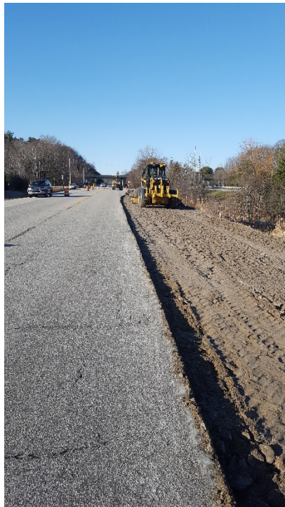
Grading base gravel in the left lane, looking south
