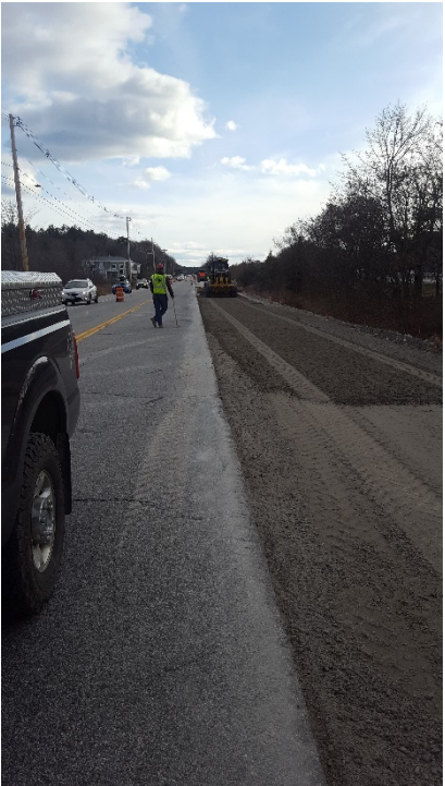
Installing crushed gravel shim in the left lane, looking south
