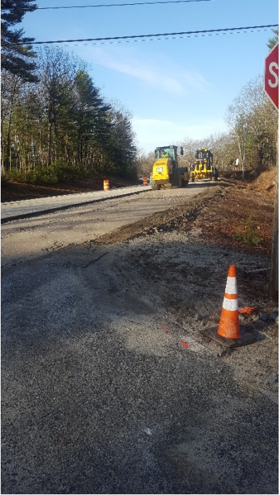
Grading base gravel in the left lane, looking south
