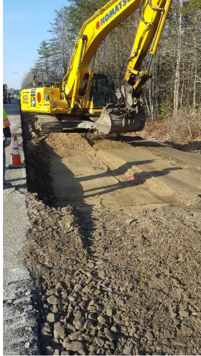
Grading subbase material in the left lane, looking south
