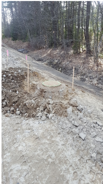
Structure prepared for adjustment in the left lane, looking south
