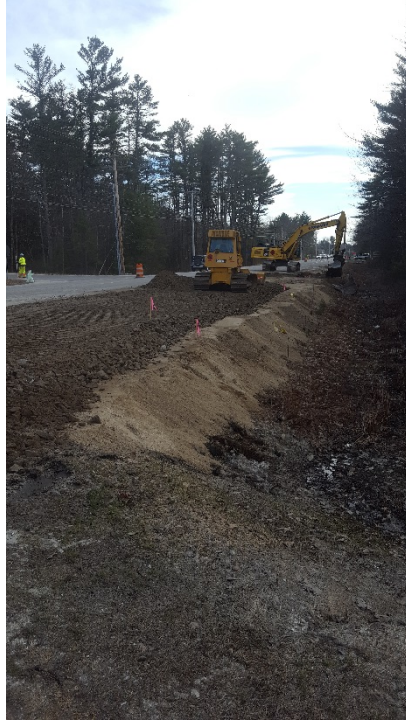
Base gravel installation in the left lane, looking south
