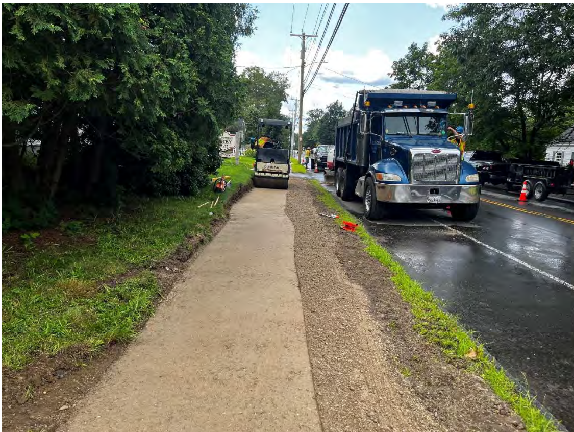
Photo 4 – Compaction of base gravel with an Ingersoll-Rand DD-24 5-ton roller.
