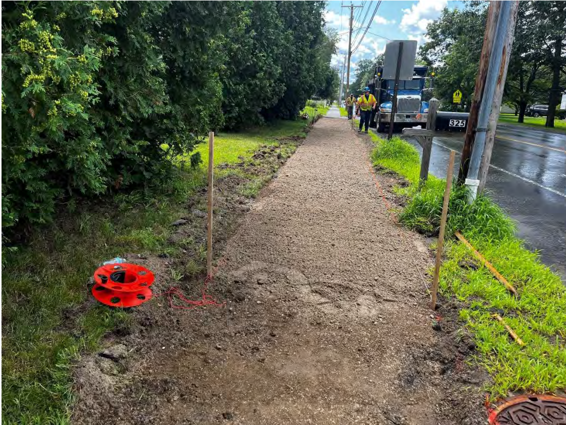
Photo 3 – String-line method set up with grade stakes for base gravel installation between 325 Main Street and 323 Main Street.
