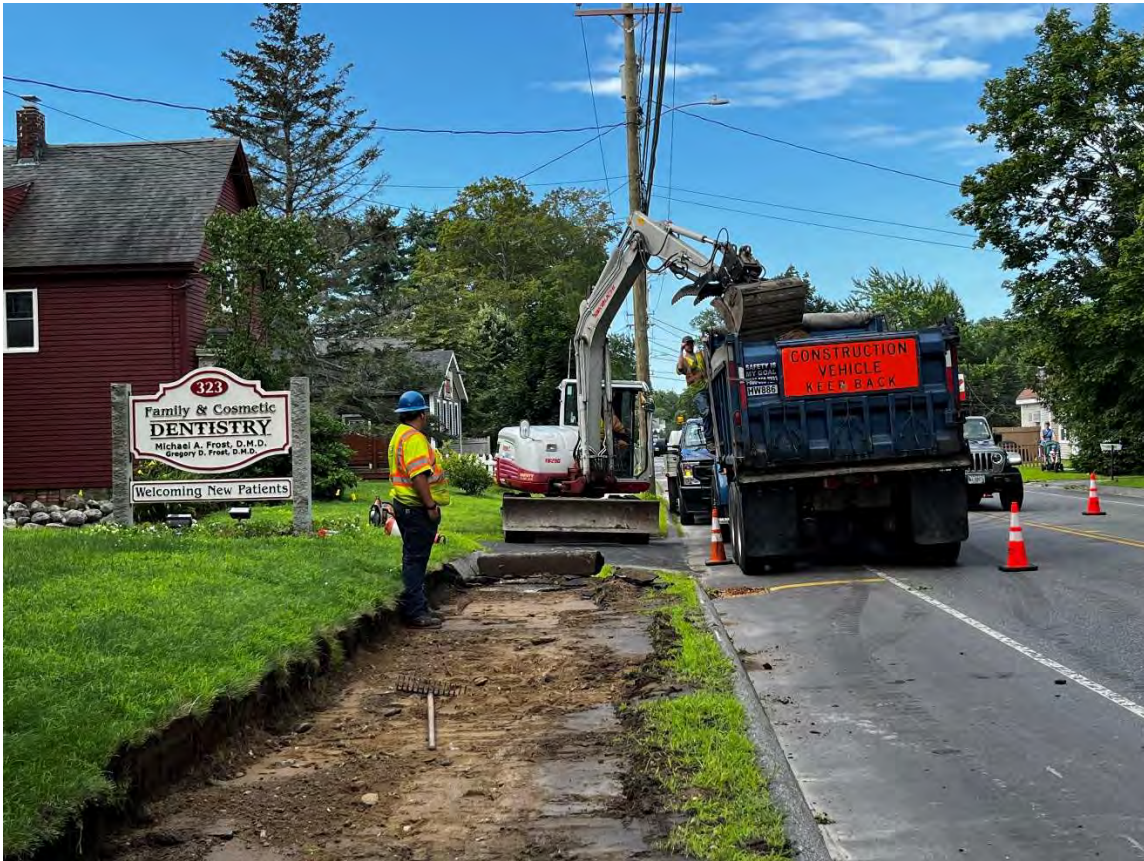
Photo 1 – Removal of existing sidewalk and behind curbing at 323 Main Street.
