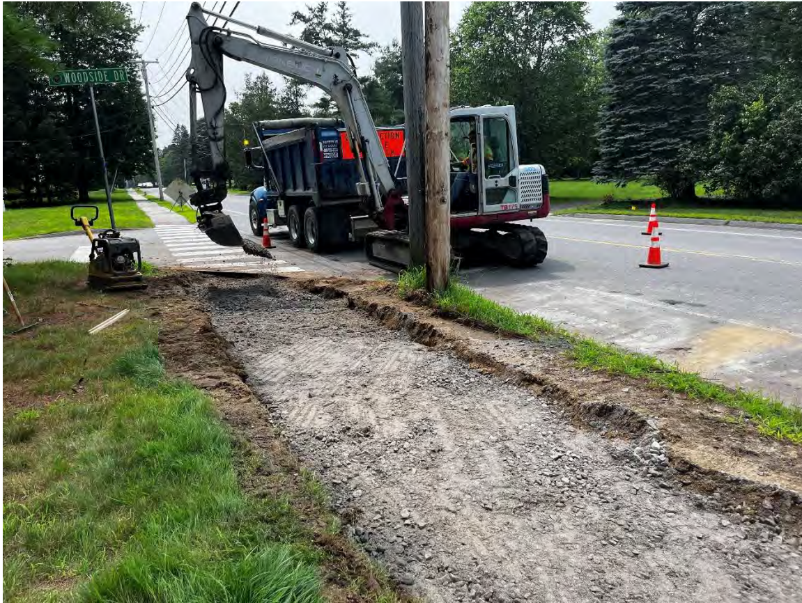
Photo 3 – Excavator operator placing subbase gravel at the apron of Woodside Drive.
