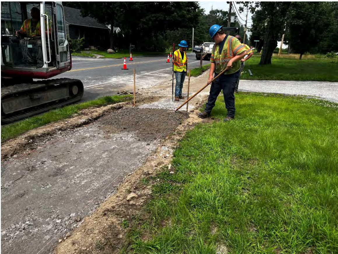
Photo 6 – Crew member raking base gravel placed by excavator.
