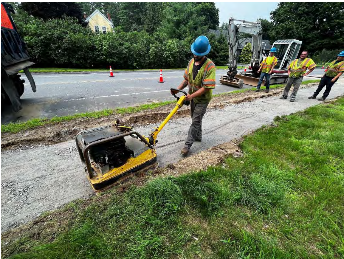
Photo 4 – Crew member compacting subbase gravels with Wacker Neuson Plate Compactor.
