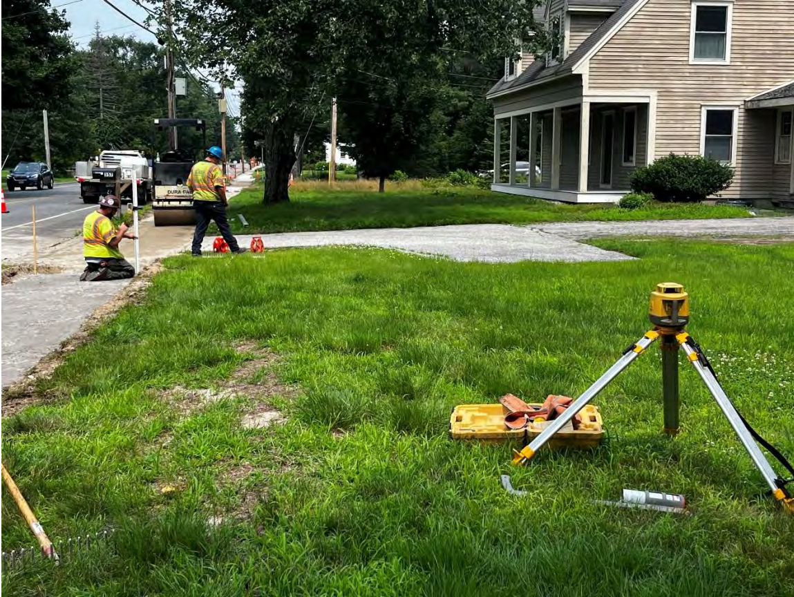
Photo 5 – Adam, foreman, using laser level to mark top of base gravel elevation for string-line method.
