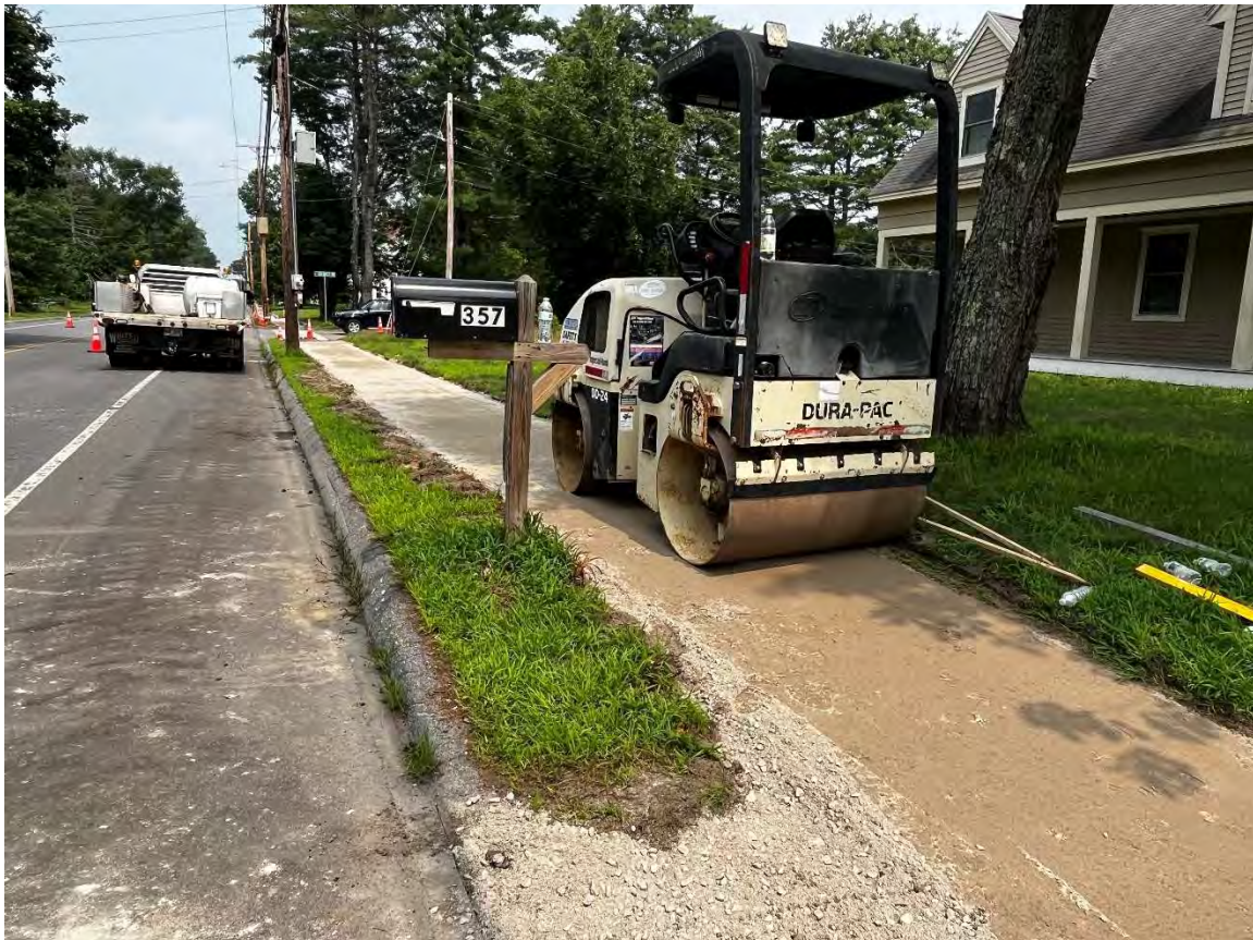
Photo 2 – Ingersoll-Rand DD-24 5-ton roller used to compact base gravels to 357 Main Street
