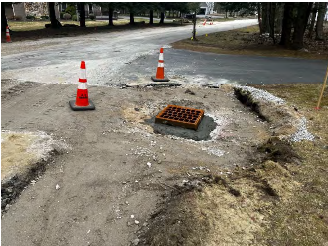
Photo 6 – Collar, frame and cover installed on CB #25. Cones directing traffic away are also pictured.
