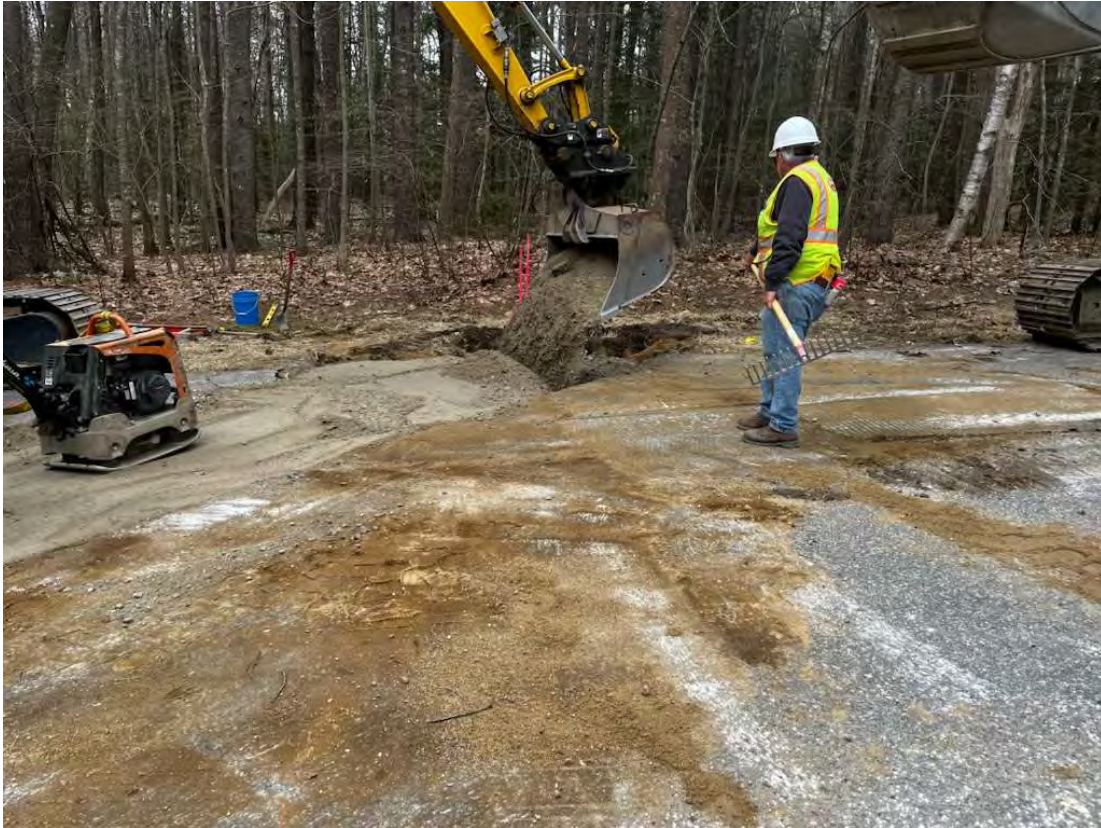
Photo 3 – CB #20 being backfilled, installed on the proposed curb line.
