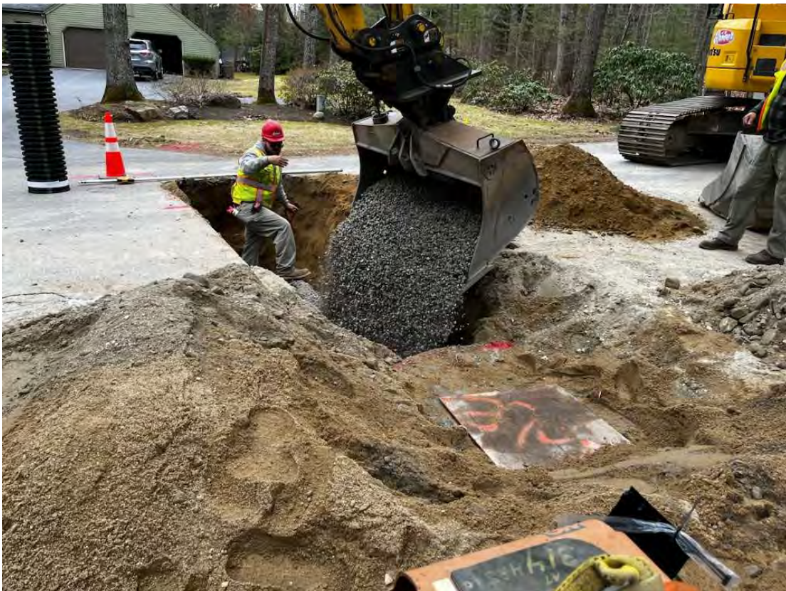
Photo 4 – Underdrain being installed to the spring line of the 12" SD between CB #24 and CB #25.
