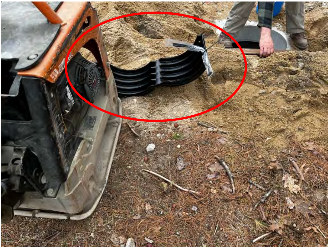
Photo 2 – 'Clamshells' (circled in red) used at joints of pipe segments.
