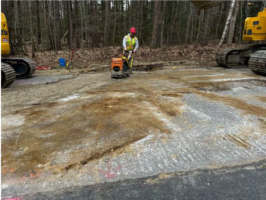
Photo 1 – Subbase in trench area compacted with plate compactor.
