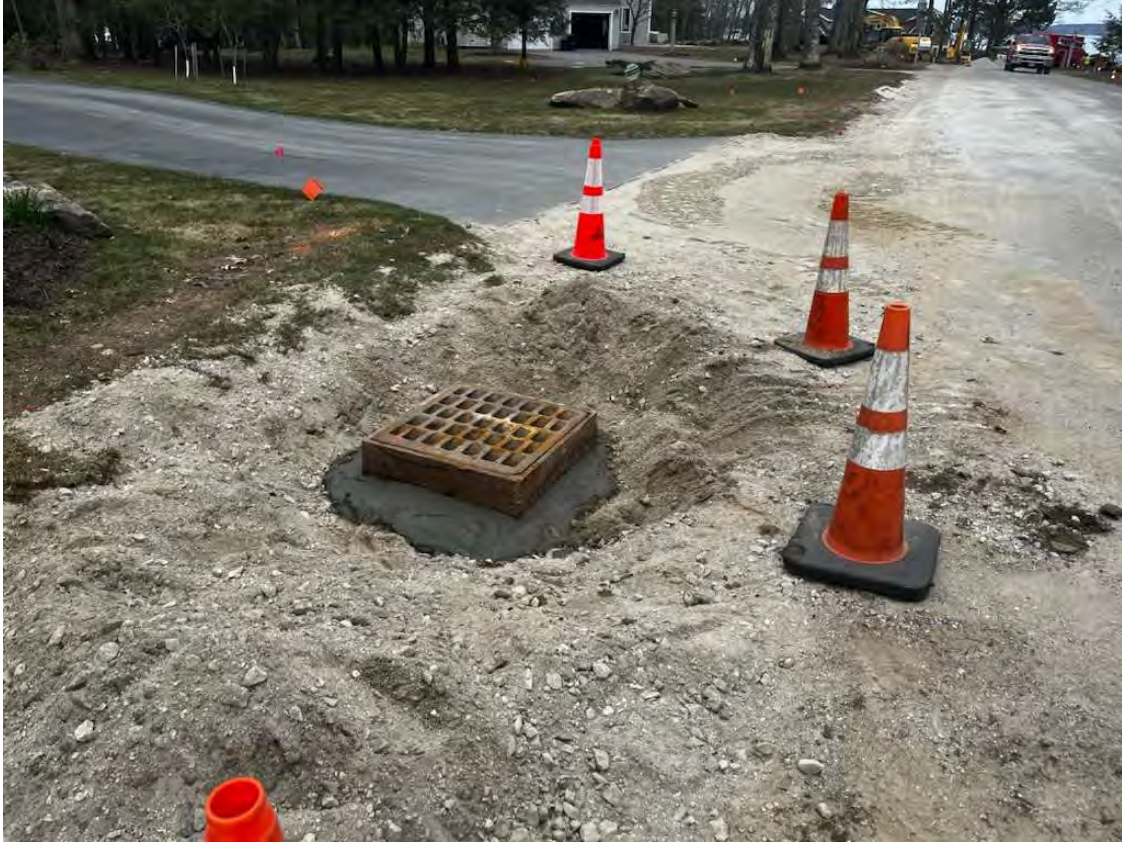
Photo 5 – Collar, frame and cover installed on CB #24. Cones directing traffic away are also pictured.
