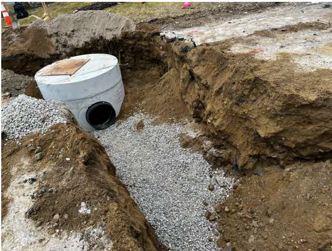
Photo 4 – \frac{3}{4} " crushed stone being placed for 15" SD pipe.
