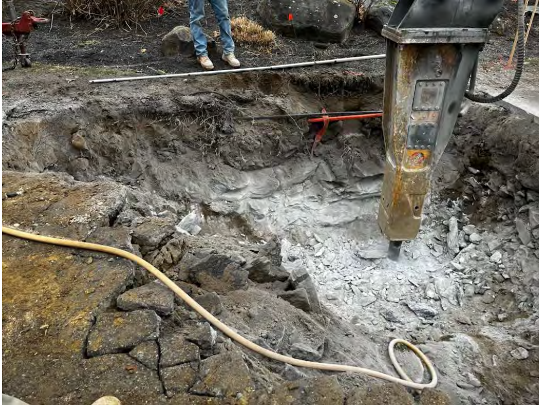
Photo 3 – Significant ledge rock in area proposed for CB #27
