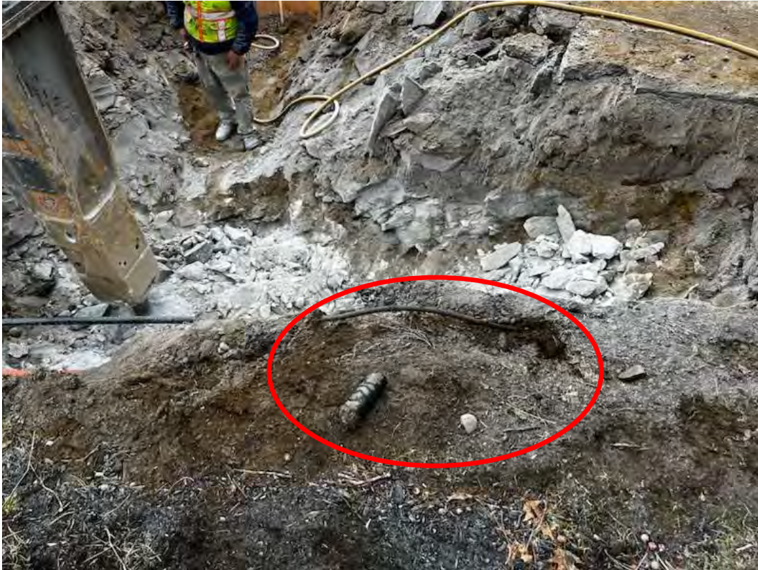
Photo 5 – Irrigation system (circled in red) damaged from excavation.
