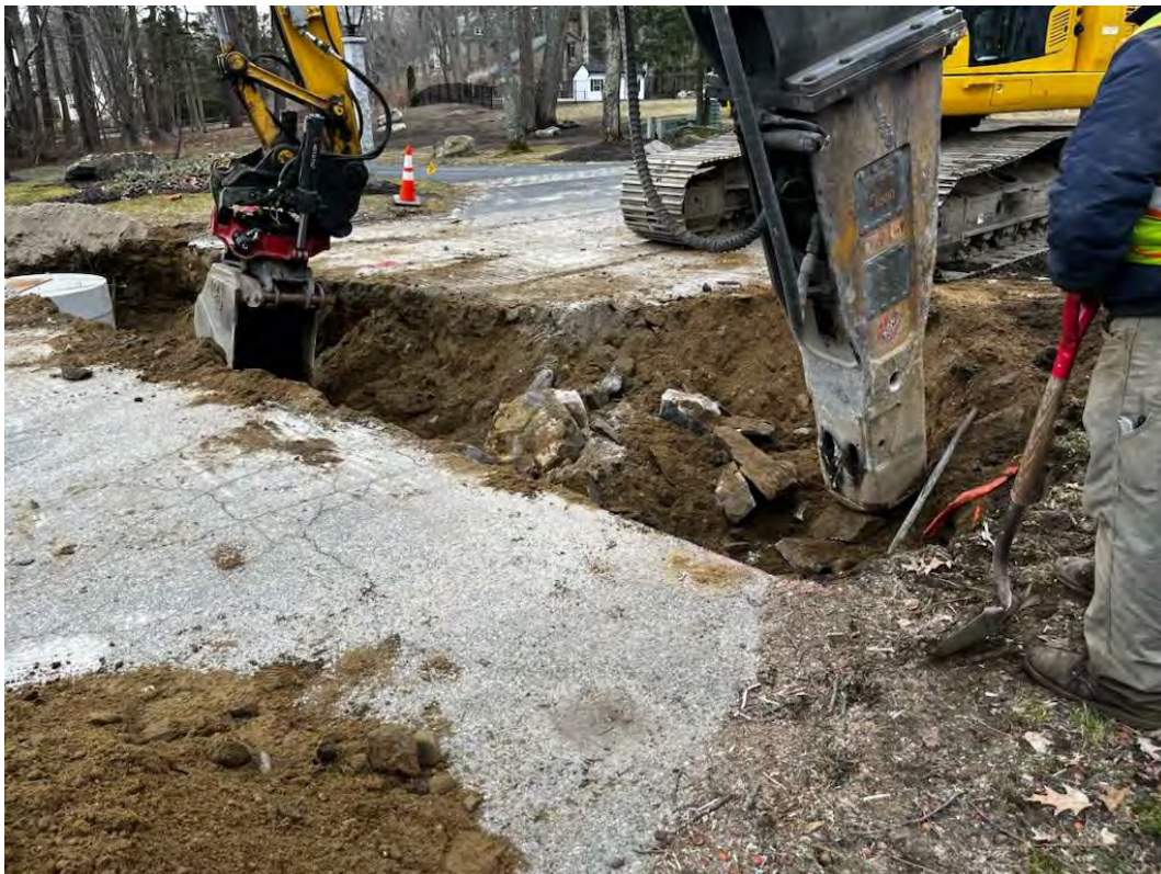
Photo 2 – Excavating trench for proposed 15" SD between CB's #27 & #28
