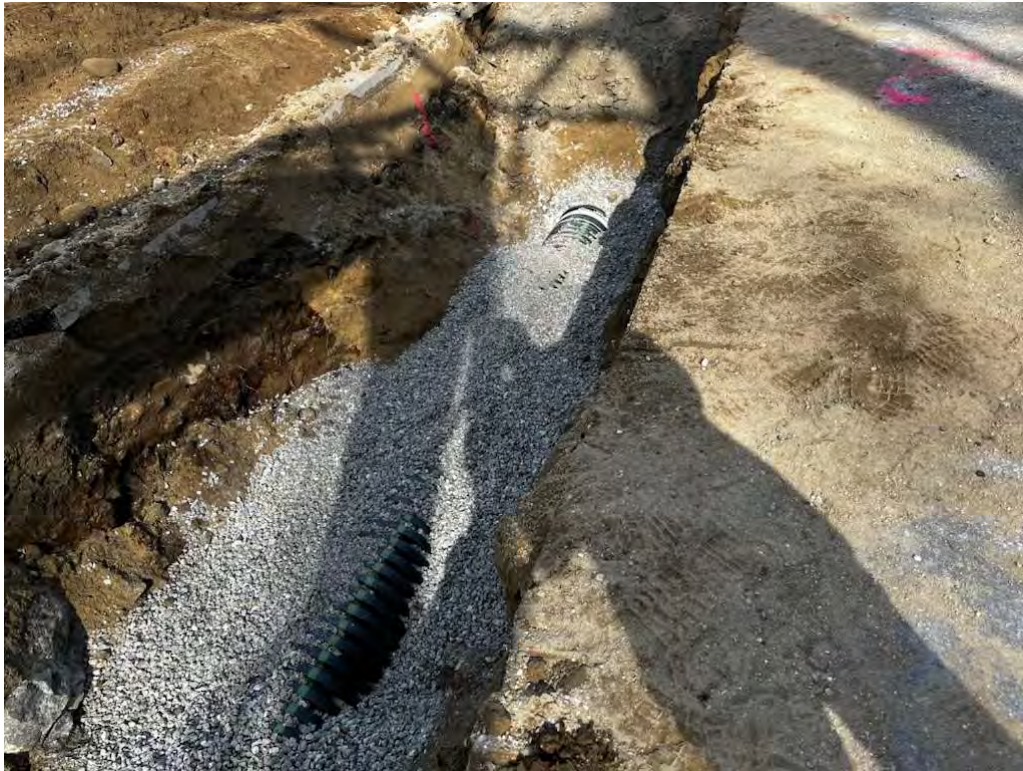
Photo 5 – Storm drain backfilled with crushed stone.
