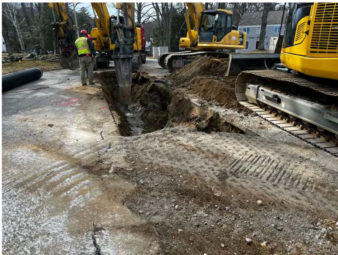
Photo 4 – Excavator with rock hammer attachment for ledge rock encountered.
