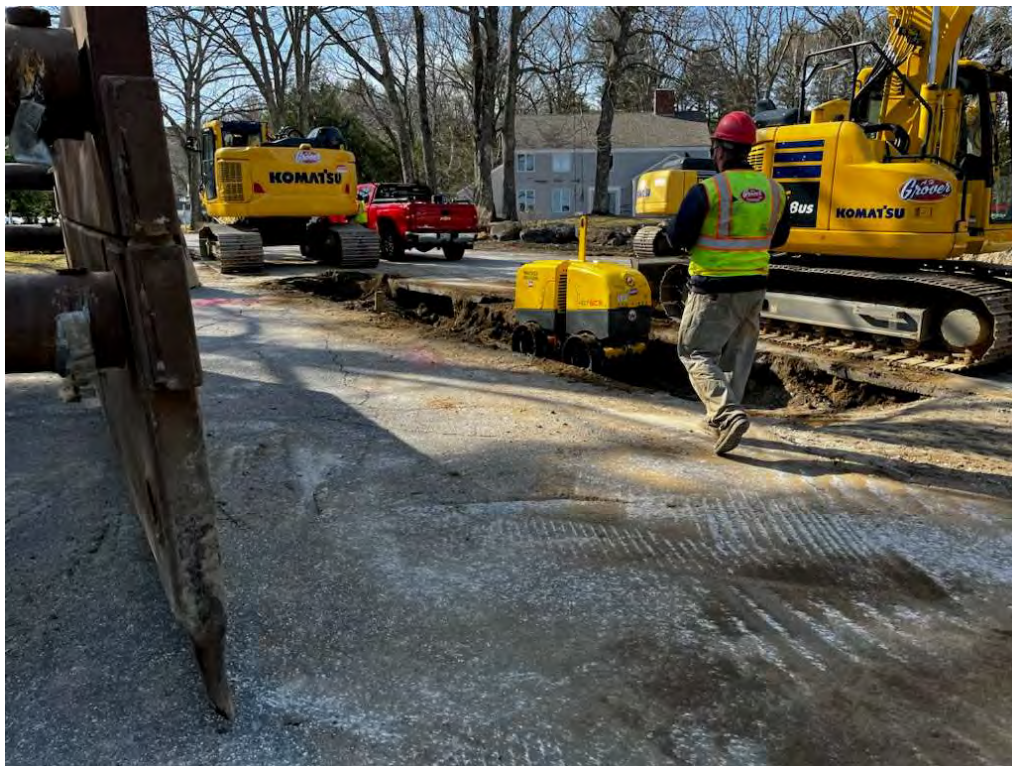
Photo 6 – Remote control Wacker Neuson compacting trench area.
