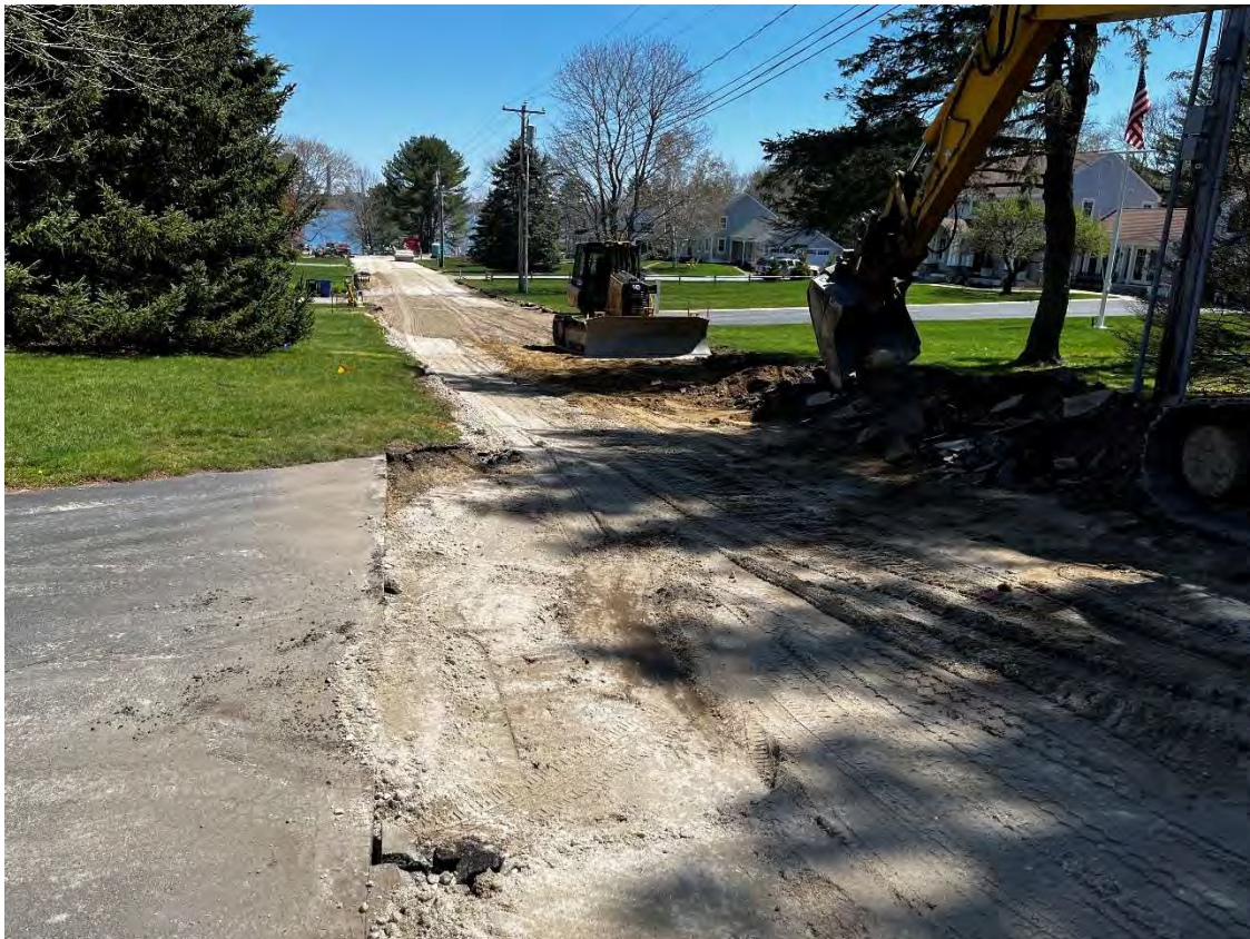
Photo 2 – Ben Grover operating Dozer to grade new surface gravels on Longmeadow Road. As can be seen in the photo, driveway of 12 Longmeadow Road has been saw cut.
