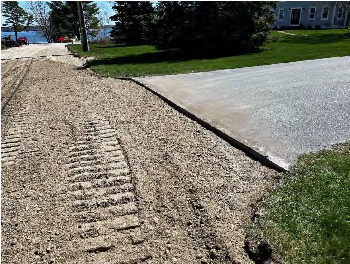
Photo 3 – Driveway of 15 Longmeadow Road saw cut.
