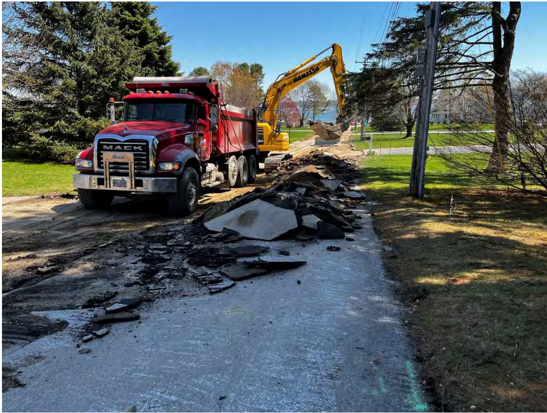
Photo 1 – Matt Grover operating the excavator to remove existing pavement.
