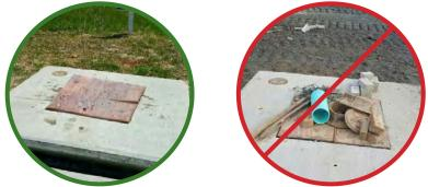
2. Final paving must be completed. Final paving ensures that paving materials will not enter and contaminate the Filterra system during the paving process, and that the plant will receive runoff from the drainage area, assisting with plant survival for the Filterra system.
