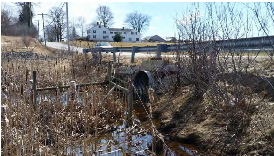
76 inch dia. Greely Road Culvert B- at Maxfield Brook – East of Site & RR Tracks
