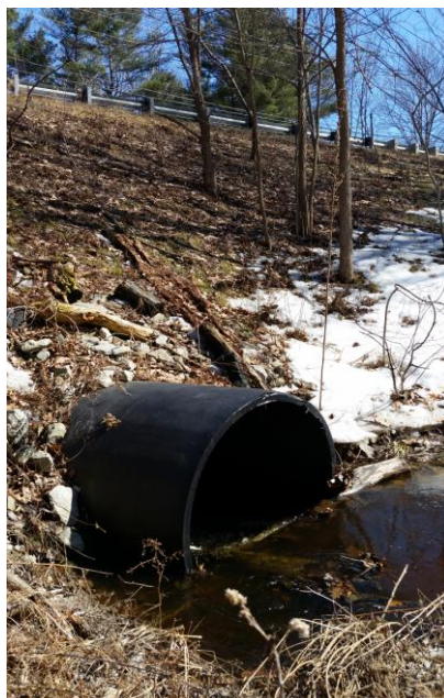
Culvert D - 48 inch HDPE inlet and embankment At Route 9 at main brook
