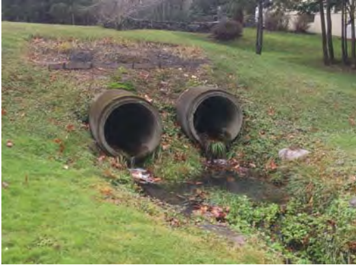
Two 30" Culverts draining to Val Halla Golf Course Below Hemlock Drive
