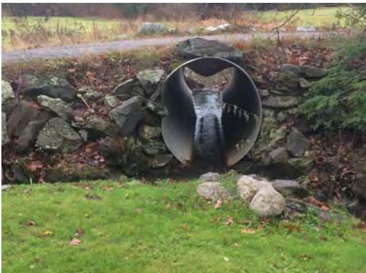
48" culvert crossing Golf Cart Path and pond storage below outlet
