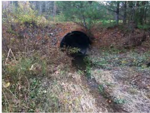
Golf Cart Path crossing Controls flow out of pond – Oval 4'X3' and 30" overflow pipe Pond 5P
