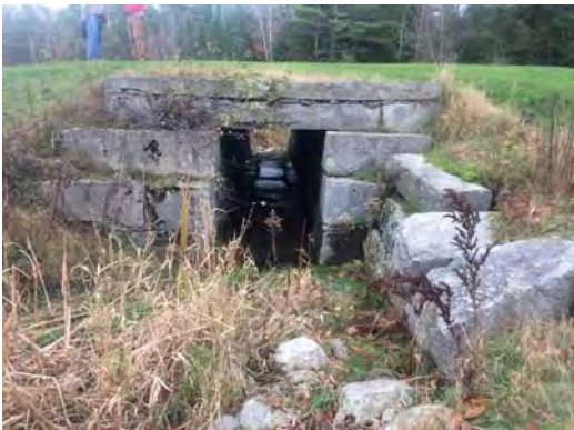
4'X6' Box Culvert under old Railroad Bed
