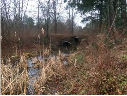
Golf Cart Path crossing Controls flow out of pond – Oval 4'X3' and 30" overflow pipe Pond 5P
