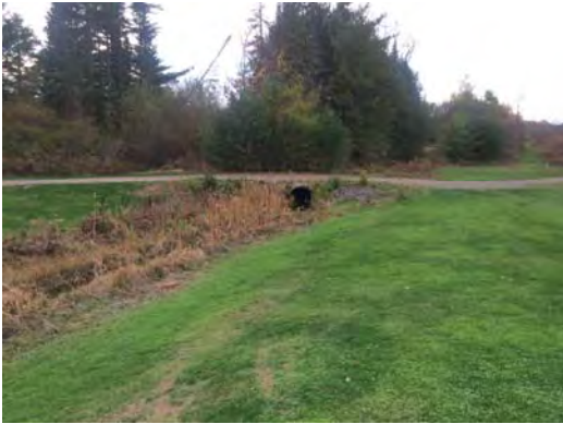
48" culvert crossing cart path outlet – Hydrocad Pond 6P
