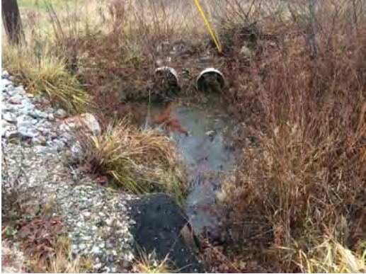
Two culverts Crossing Tuttle Road 30" & 24" (below site) – Hydrocad Pond 1P
