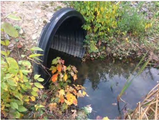
48" culvert crossing cart path inlet – Hydrocad Pond 6P
