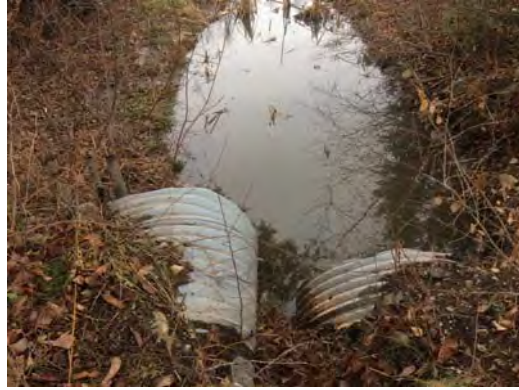
Golf Cart Path crossing Controls flow out of pond – Oval 4'X3' and 30" overflow pipe Pond 5P
