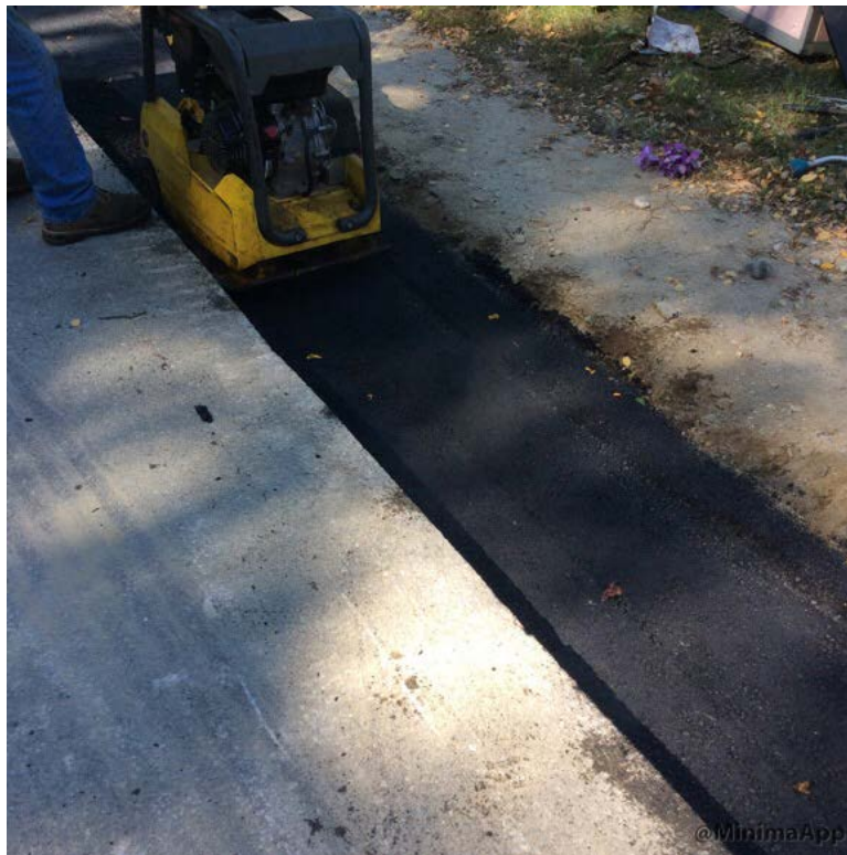
Compacting first lift of 12.5mm HMA with plate wacker.
