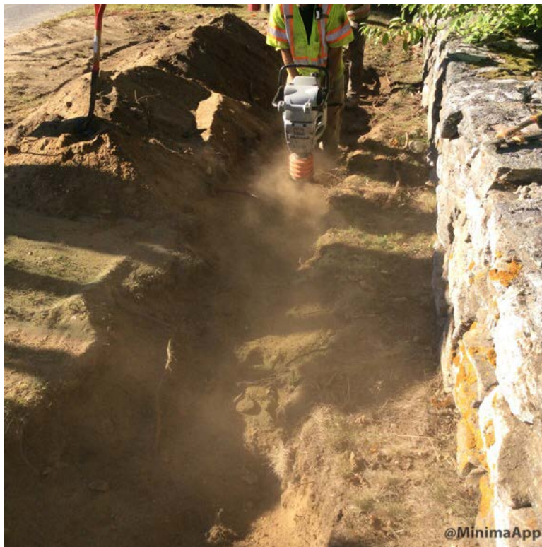
Compacting backfill with jumping jack near Deans Way.
