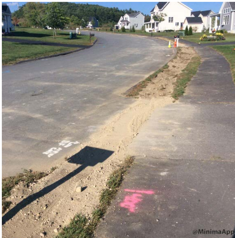
Driveway crossing at #3 Castlerock Drive backfilled.
