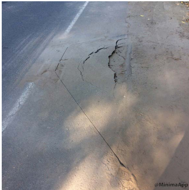
Failed pavement section on Skillin Road sawcut.
