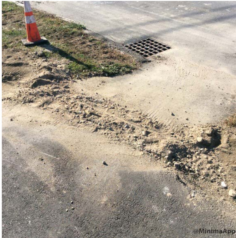
Sidewalk crossing backfilled on Castlerock Drive.
