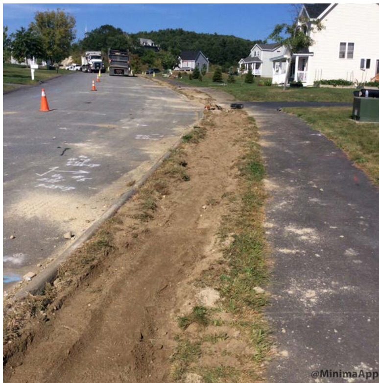
Trench in esplanade backfilled.
