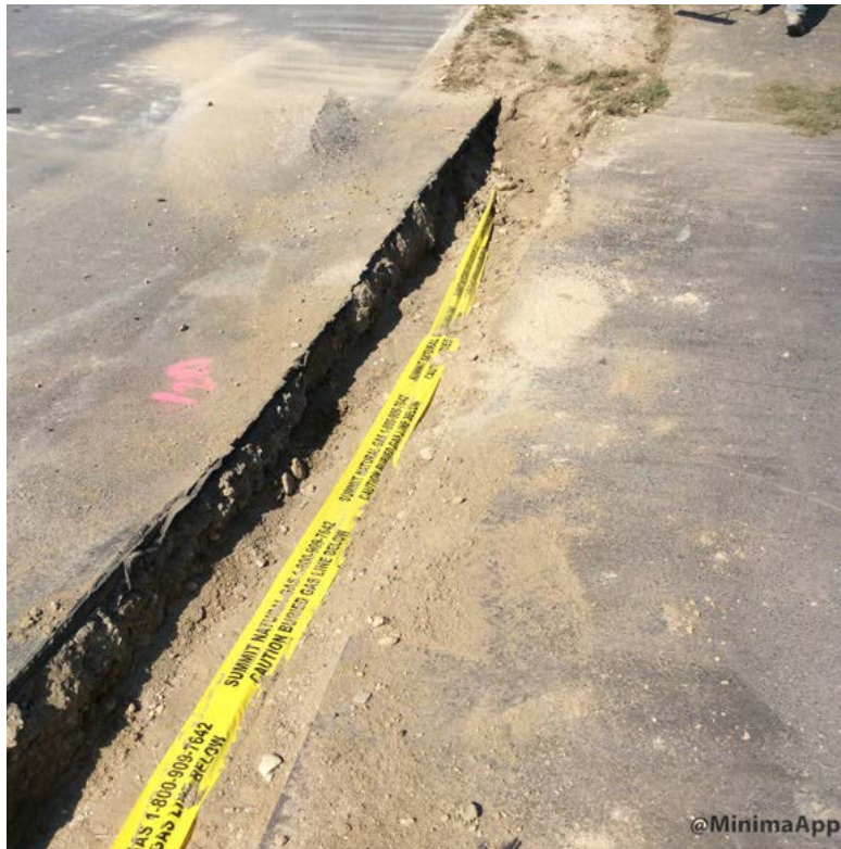
Backfill compacted and warning tape placed in driveway crossing on Castlerock Drive.
