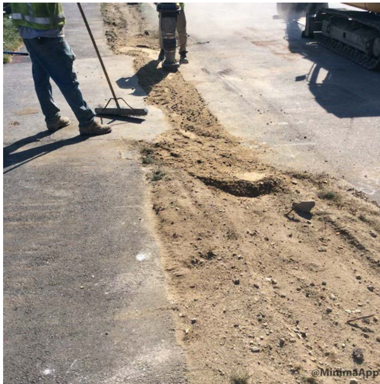
Compacting backfill at driveway crossing on Castlerock Drive.
