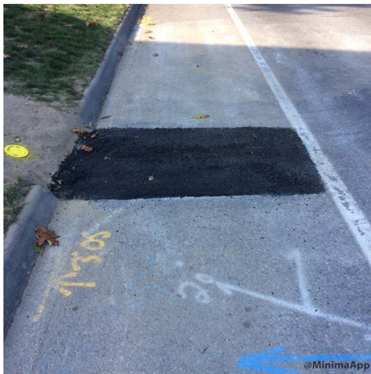
Cold patch placed in longitudinal trench on route 88.
