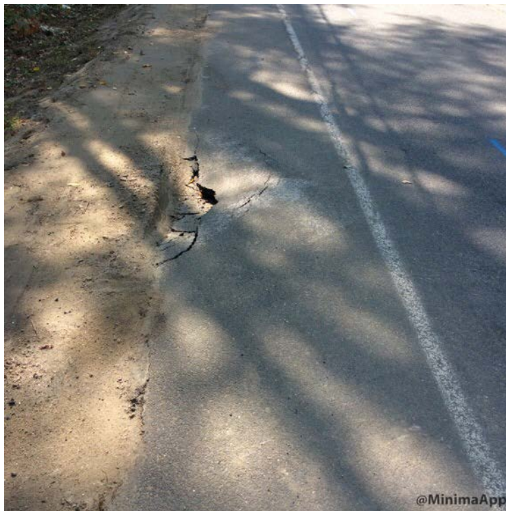
Failed section of pavement on Skillin Road
