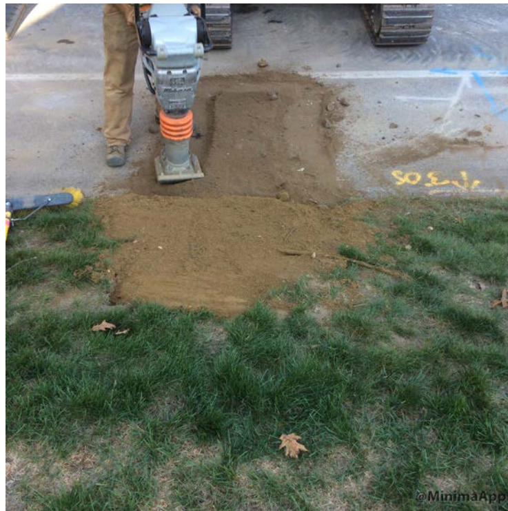
Compacting longitudinal trench on route 88
