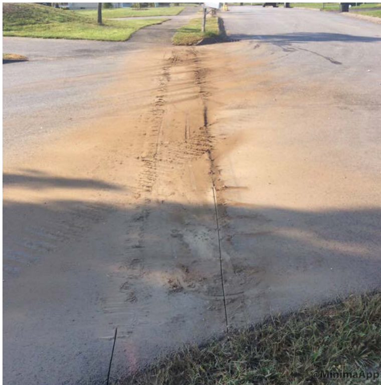
Pavement sawcut for roadway crossing trench on Castlerock Drive.
