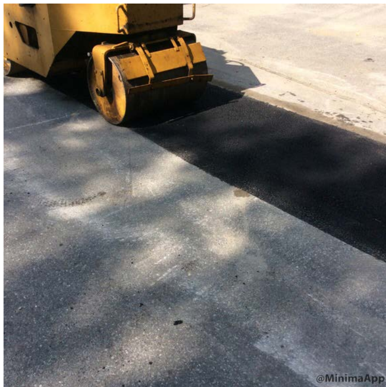
Compacting final lift of 12.5mm HMA with 3 ton vibratory roller
