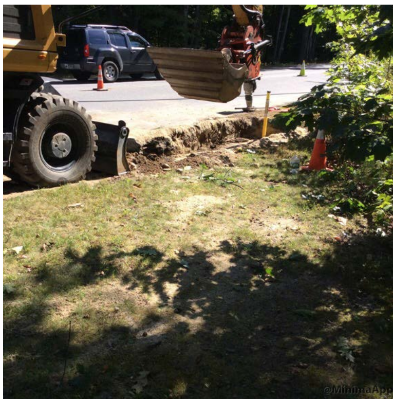
Backfilling excavated area after purging gas main.
