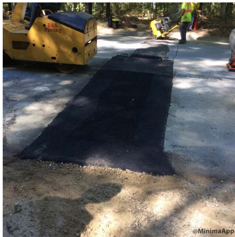
Compacting 12.5mm HMA at roadway crossing trench.
