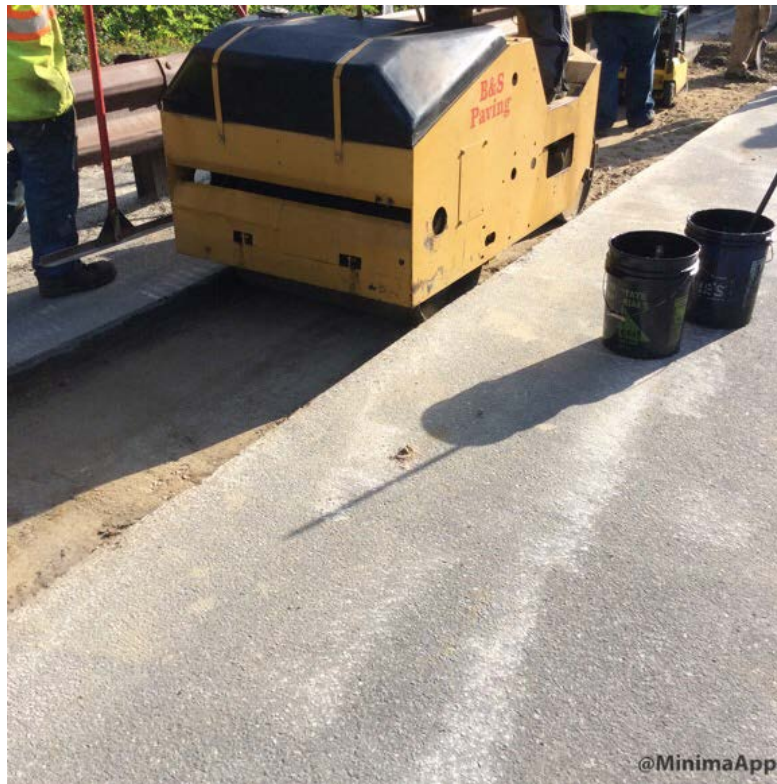
Compacting gravel trench with 3 ton vibratory roller.
