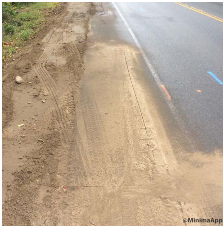
Pavement sawcut on east bound shoulder
