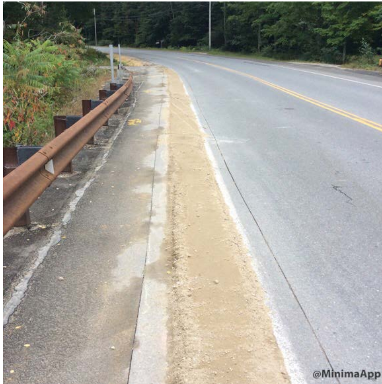
Gravel trench brought to approximate roadway grade.
