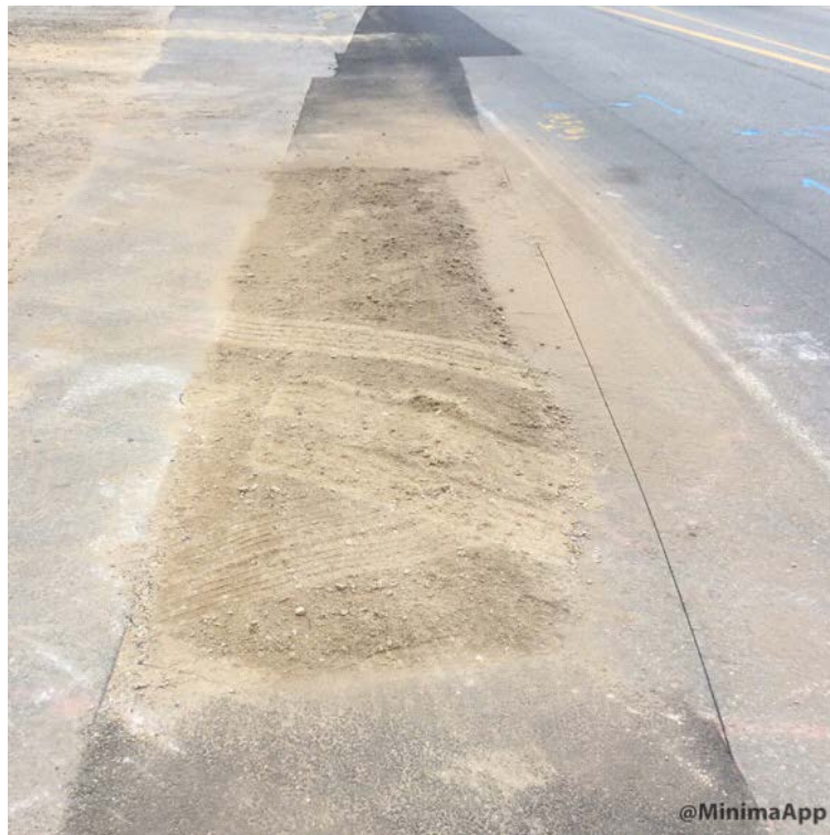
Gravel trench near Copp Motors backfilled.
