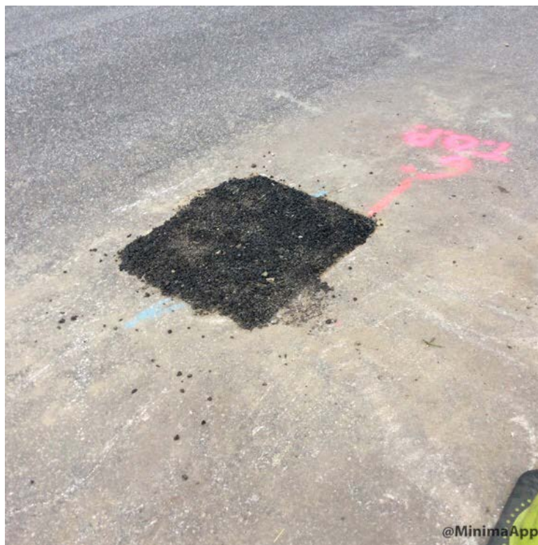
Cold patch in pothole.
