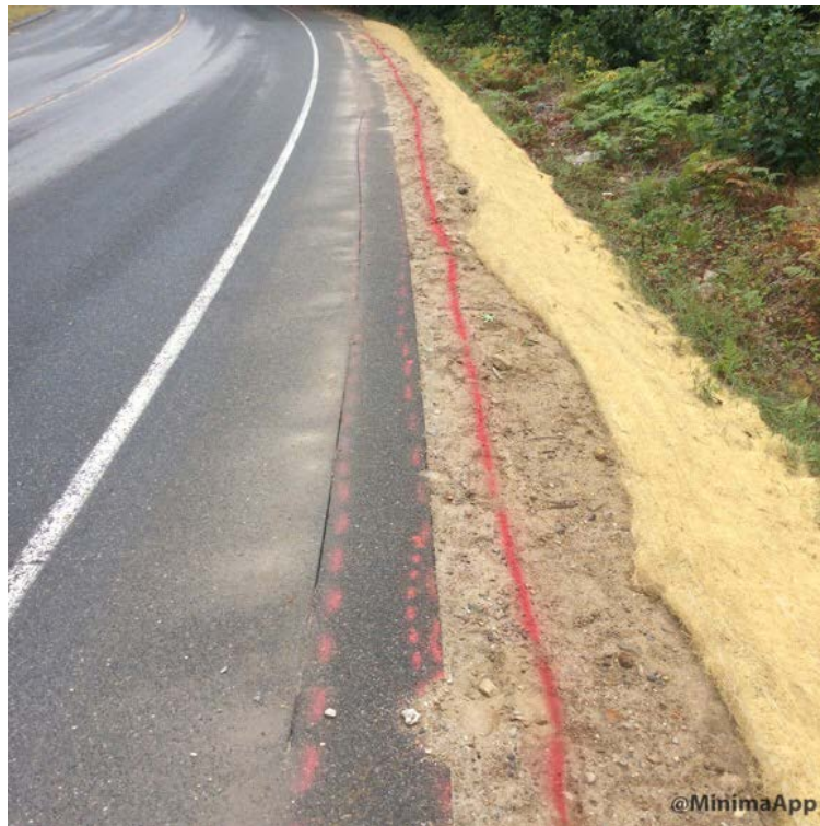
Layout of shoulder trench near large culvert.
