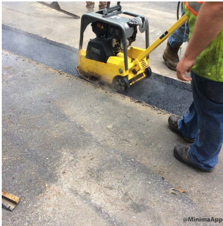
Compacting first lift in driveway trench
