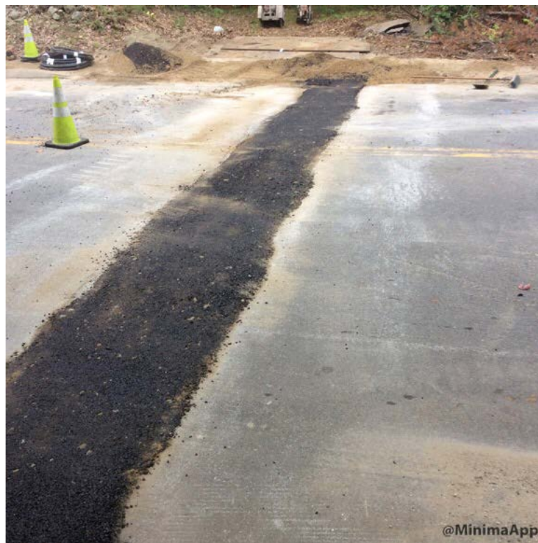
Cold patch placed in roadway crossing trench
