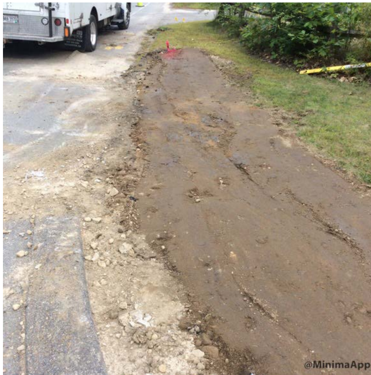
Compacted backfill at the intersection of Blanchard and Skillin
