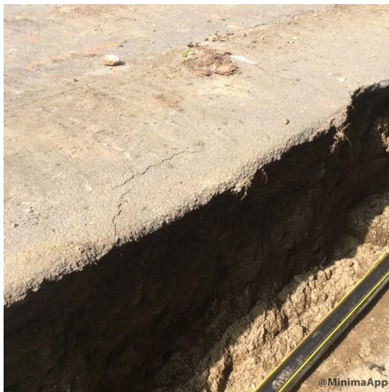
Roadway undermine due to trench excavation
