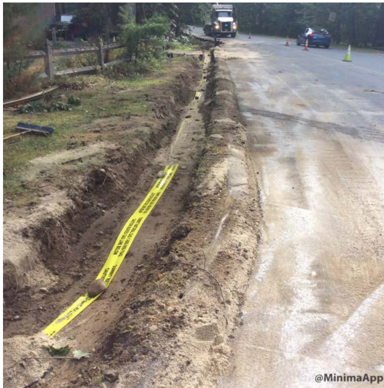
Backfill compacted and warning tape placed in trench.
