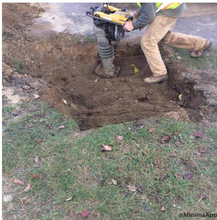
Compacting backfill in trench at vegetated island.
