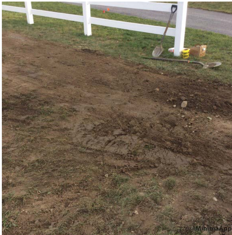
Trench on house side backfilled.
