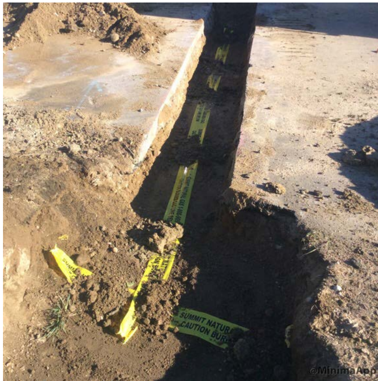
Warning tape placed in trench.
