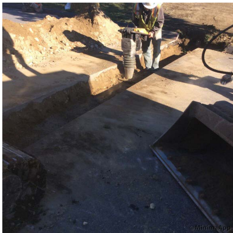
Compacting backfill with jumping jack.
