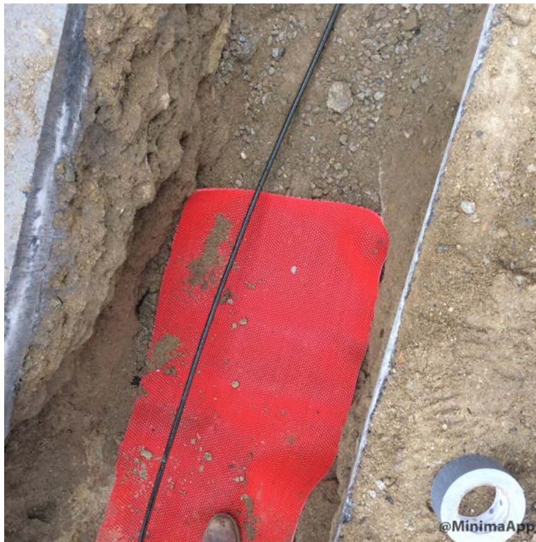
Rock shield placed between gas service and underdrain
