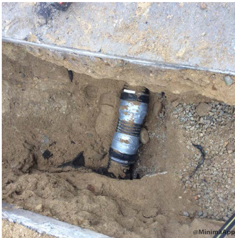
Repaired underdrain at 69 Skillin Rd.
