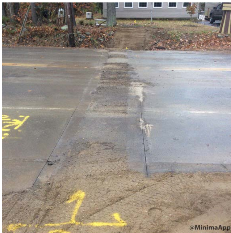
Trench backfilled with pavement cutbacks.
