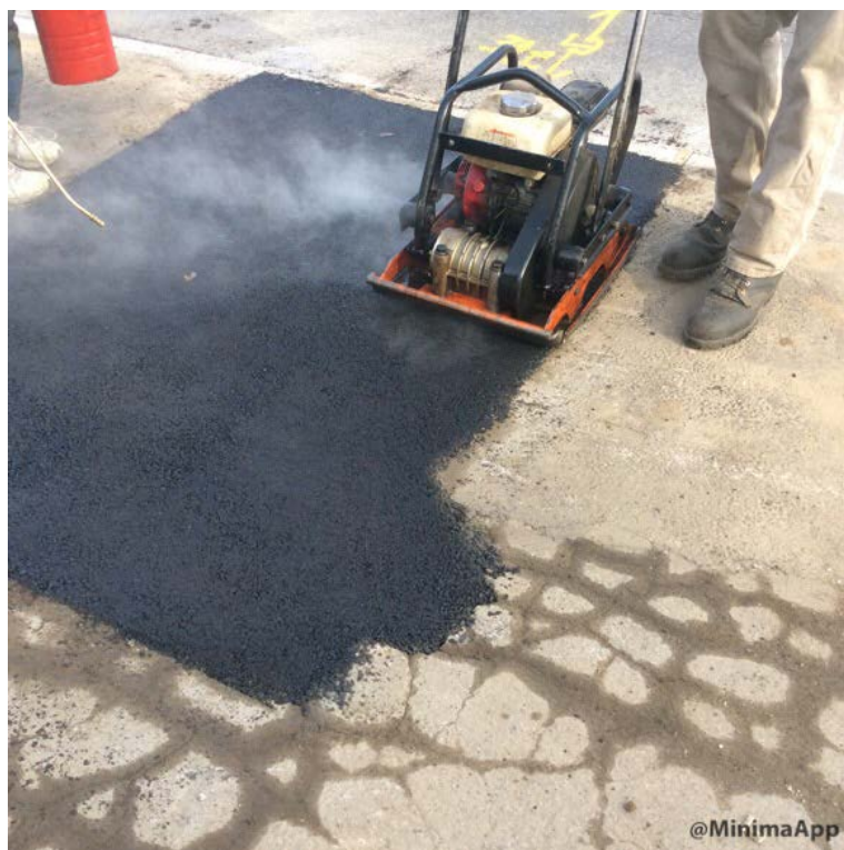
Compacting HMA with plate wacker.
