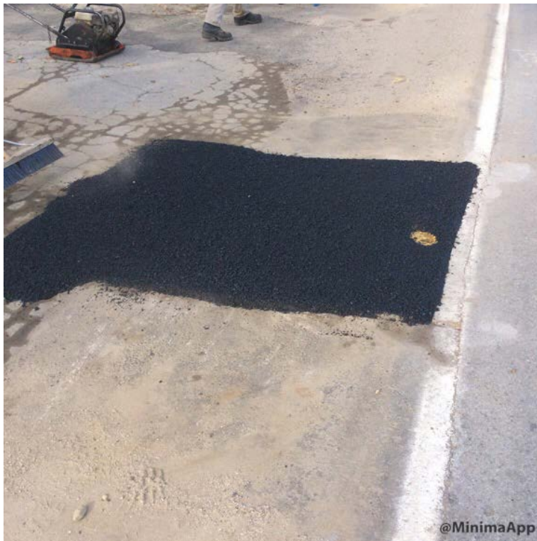
Final lift of 9.5mm HMA placed.
