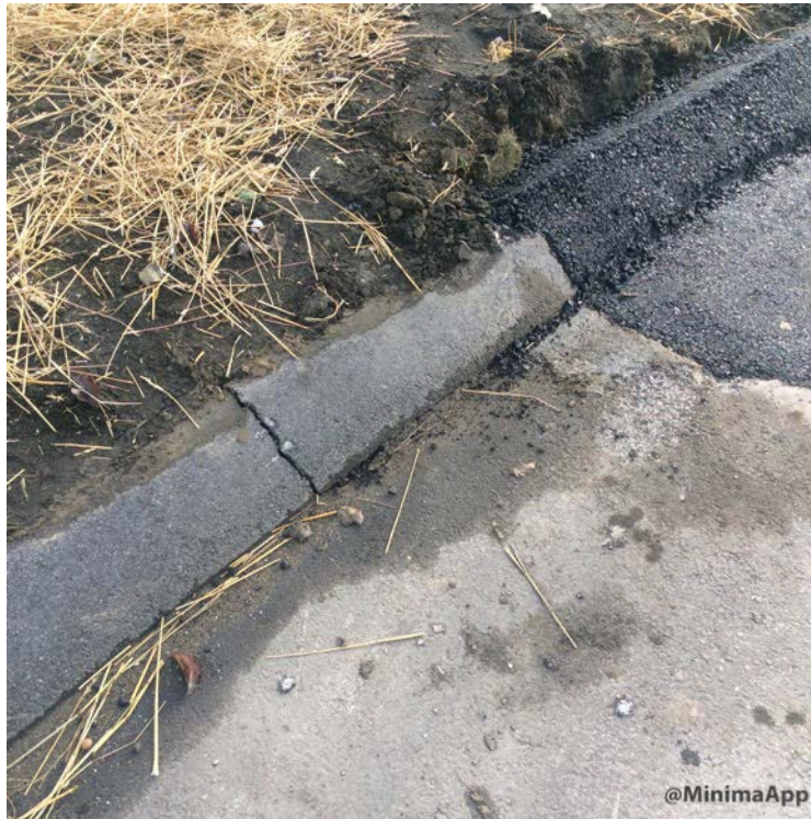
Damaged curb that was not removed prior to rebuilding curb.
