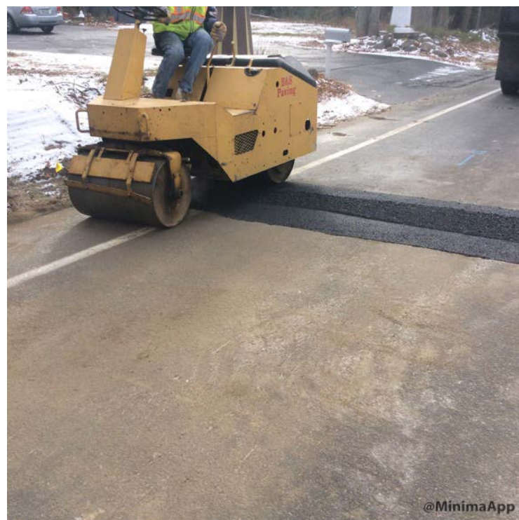
Compacting final lift of 12.5mm HMA at 69 Skillin Road.
