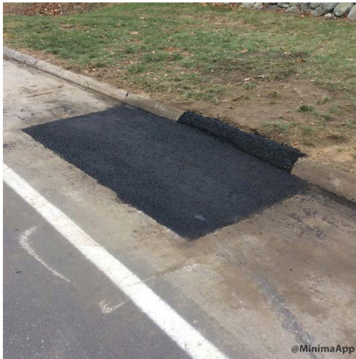
Completed trench patch in westbound lane and hand built curb at 20 Blanchard Road.
