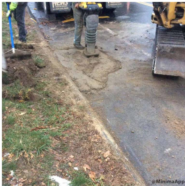
Compacting backfill on westbound lane side.
