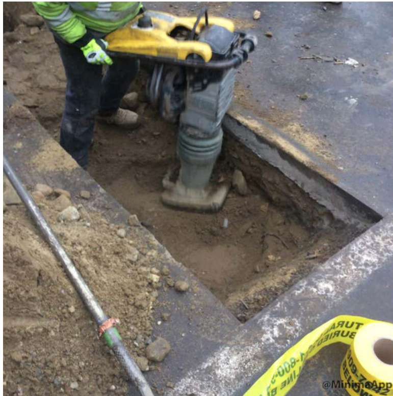
Compacting backfill in trench on eastbound lane side.
