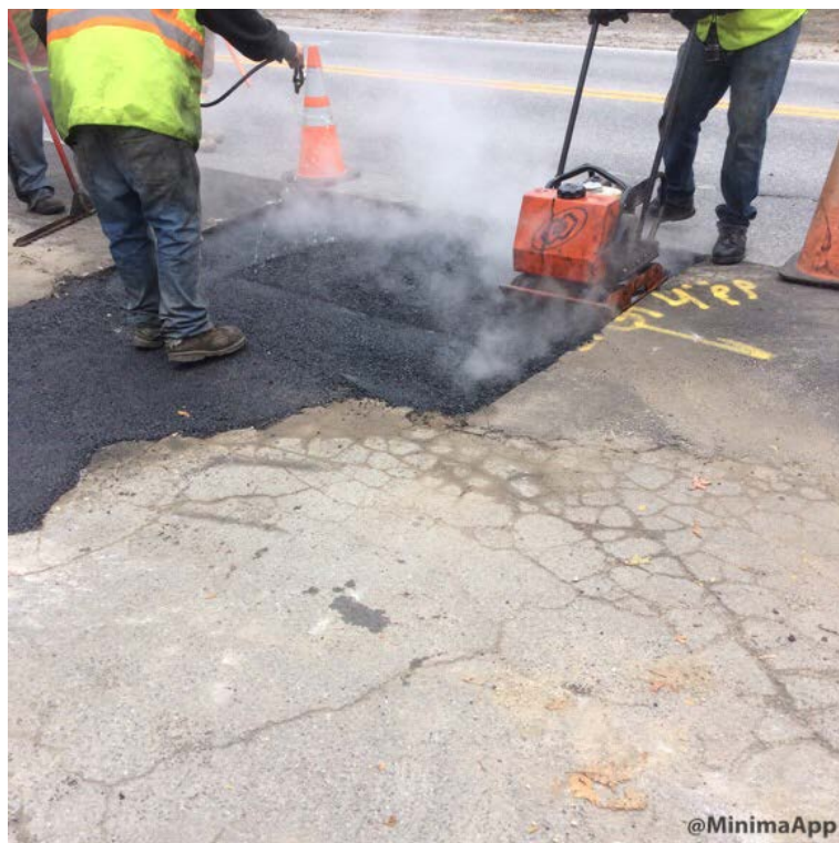
Compacting longitudinal patch at 194 Gray Road with plate wacker.
