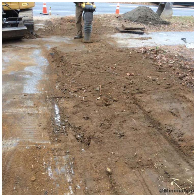
Compacting backfill with jumping jack.
