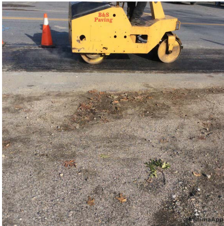
Compacting 12.5mm HMA with roller at Copp Motors
