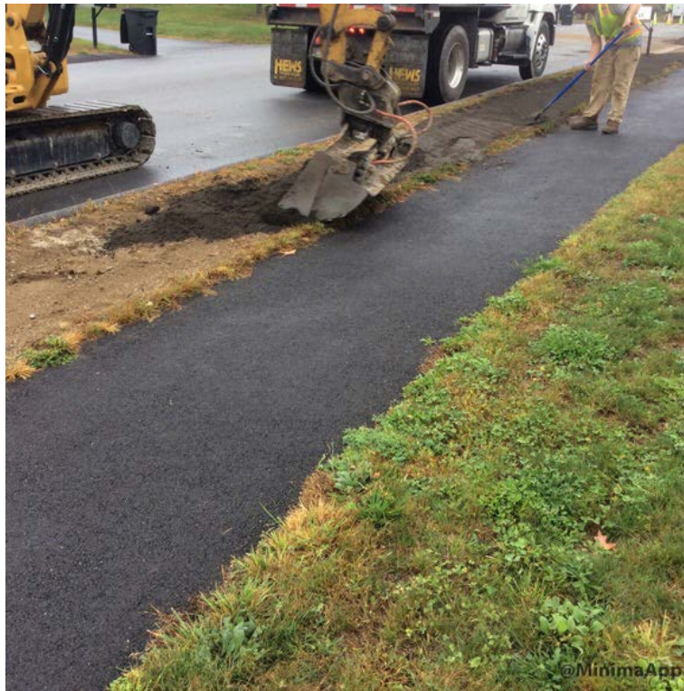
Placing loam in esplanade.
