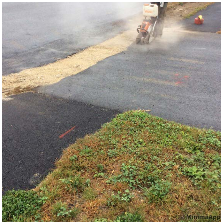
Saw cutting driveway crossing trench.
