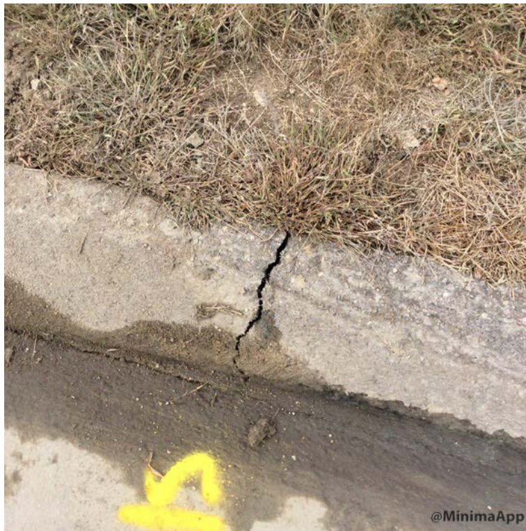
Cracking on curb on Castle Rock Dr.
