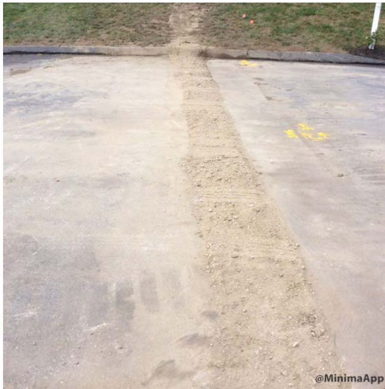
Roadway crossing trench backfilled.
