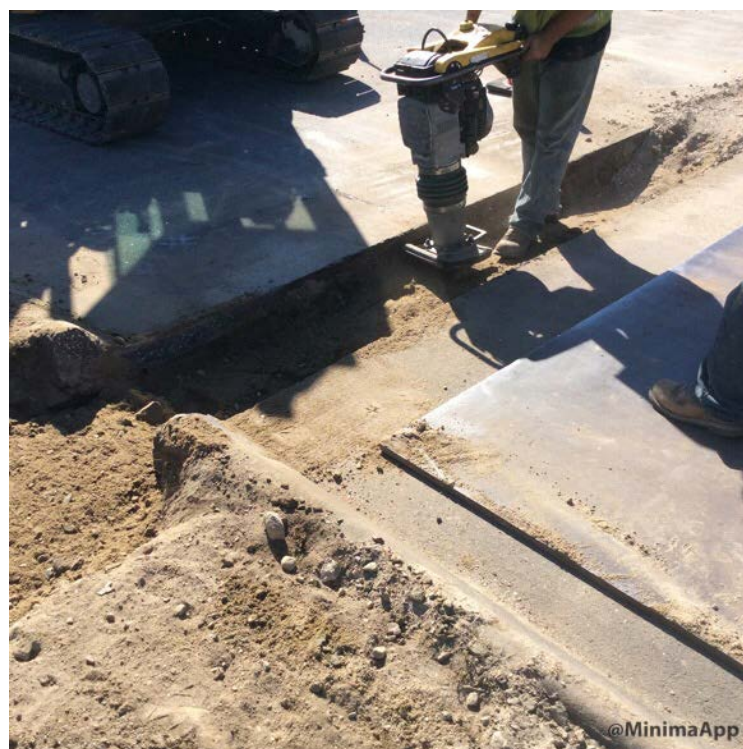
Compacting backfill on Castlerock.
