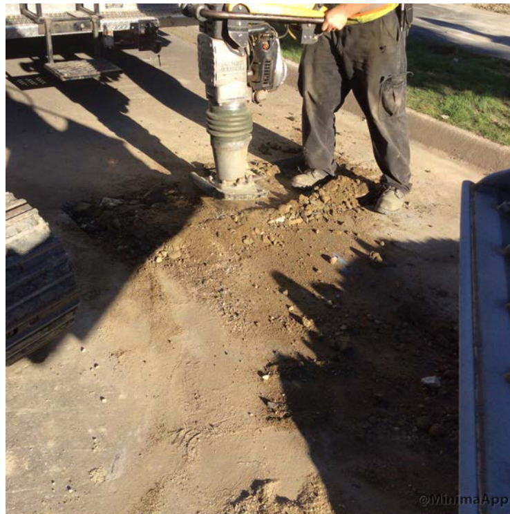
Compacting backfill in roadway on Wyman Way
