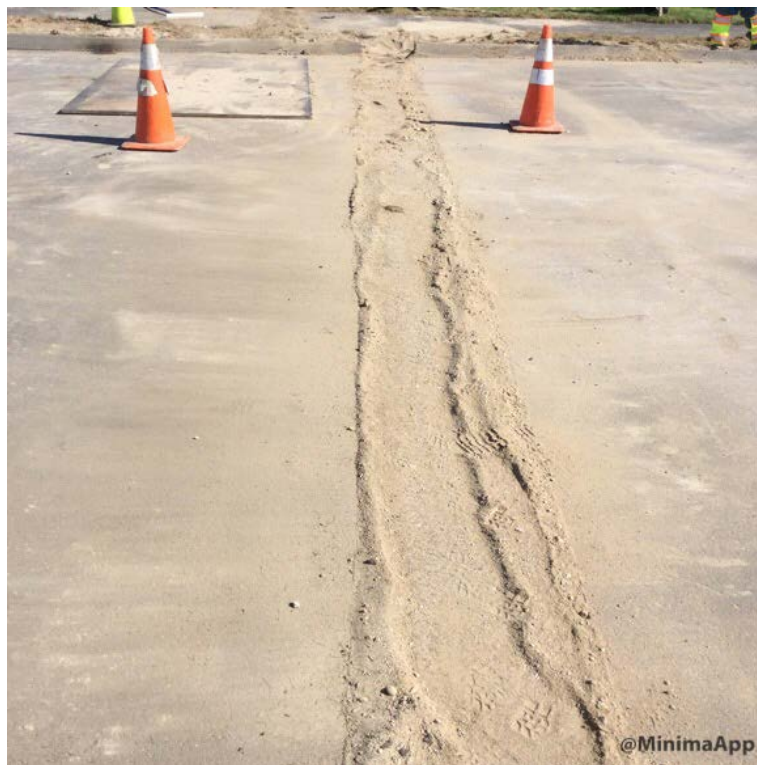
Trench backfilled and gravel compacted on Castlerock.
