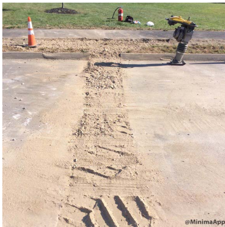
Trench backfilled and compacted on Castlerock Drive.
