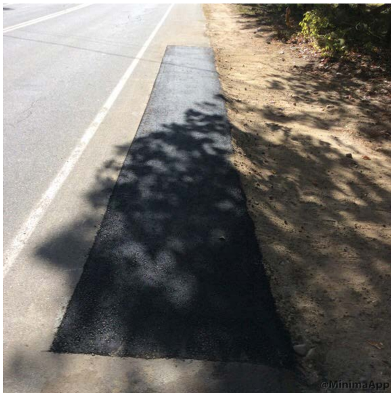
Completed roadway shoulder trench patch on Skillin Road.
