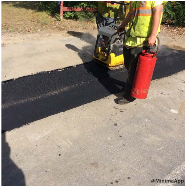
Crew compacting first lift of 12.5mm HMA.
