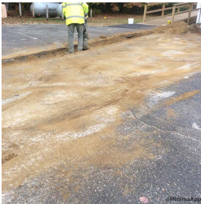
Comparing backfill with jumping jack.
