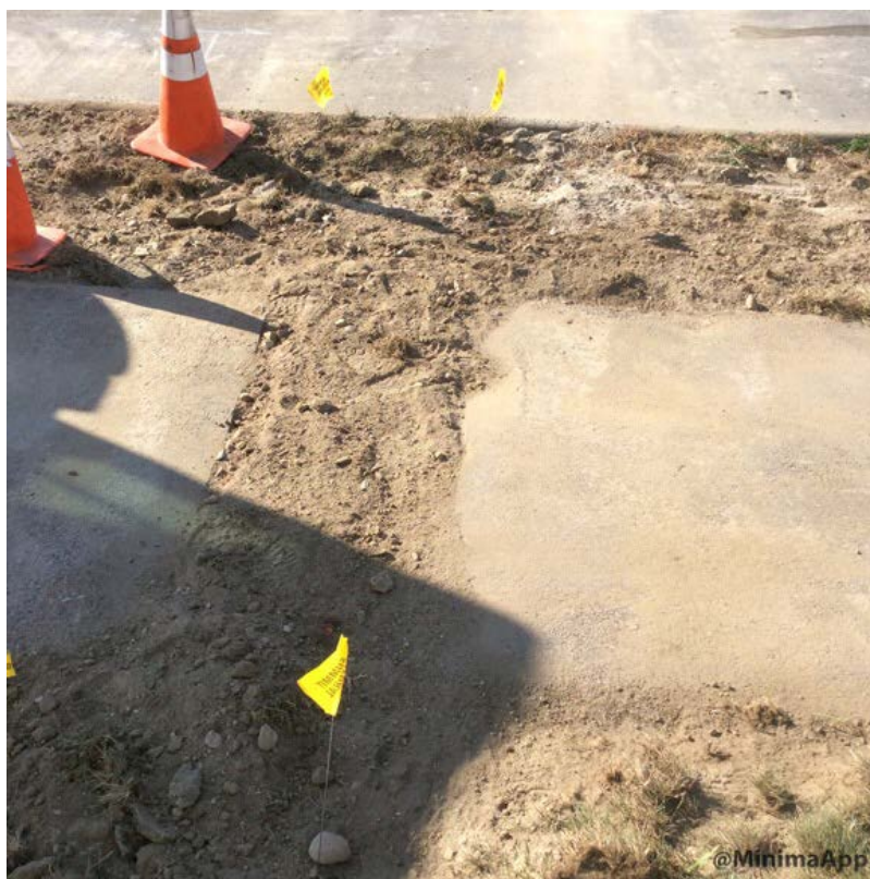
Sidewalk crossing trench backfilled.
