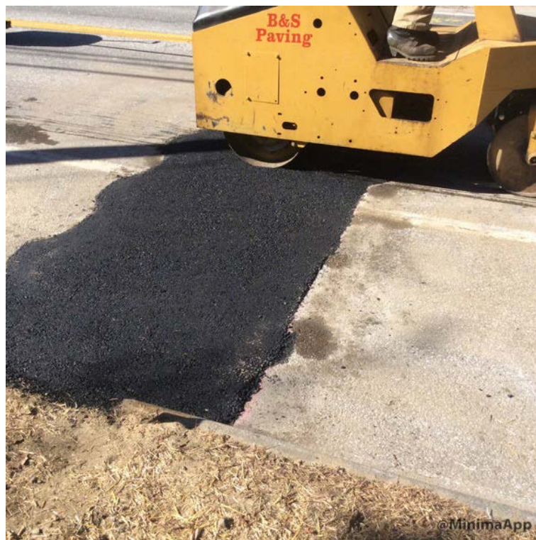
Compacting 12.5mm HMA on Main Street with 3 ton roller.
