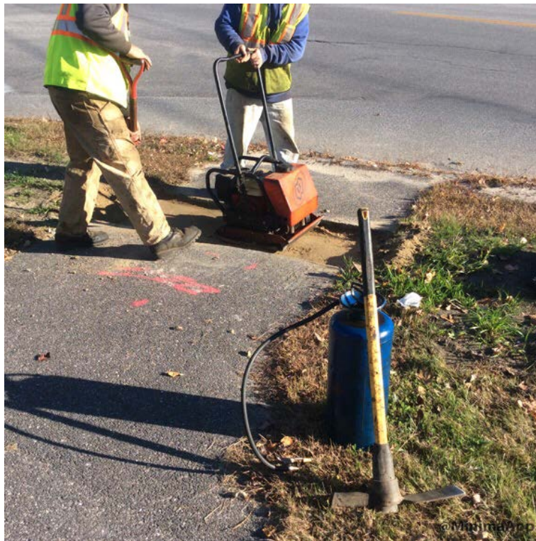
Compacting gravel for sidewalk trench.
