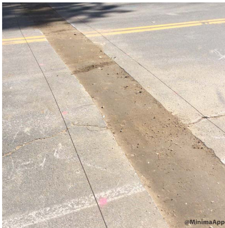
Roadway crossing trench backfilled and compacted on Skillin Road.
