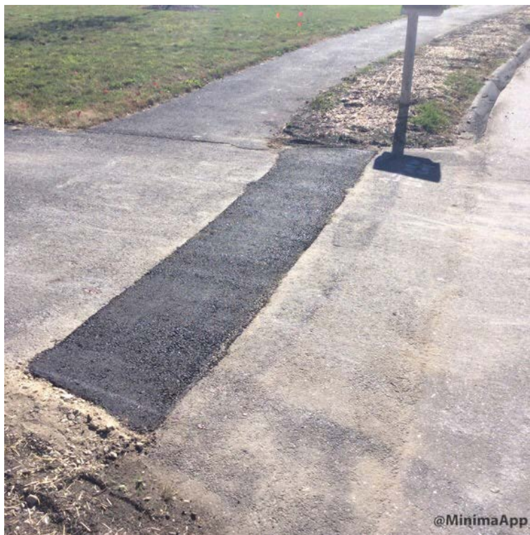
Completed driveway crossing trench.
