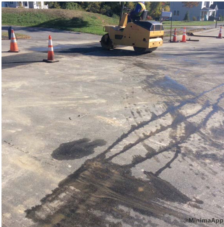
Compacting final lift of roadway crossing trench with 3 ton roller.
