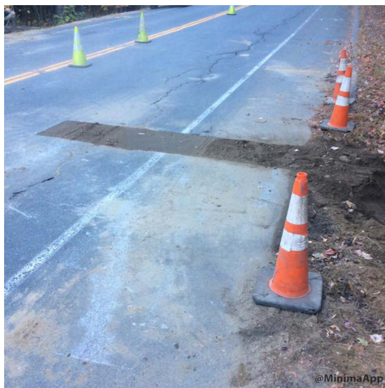
Westbound lane trench backfilled and compacted.
