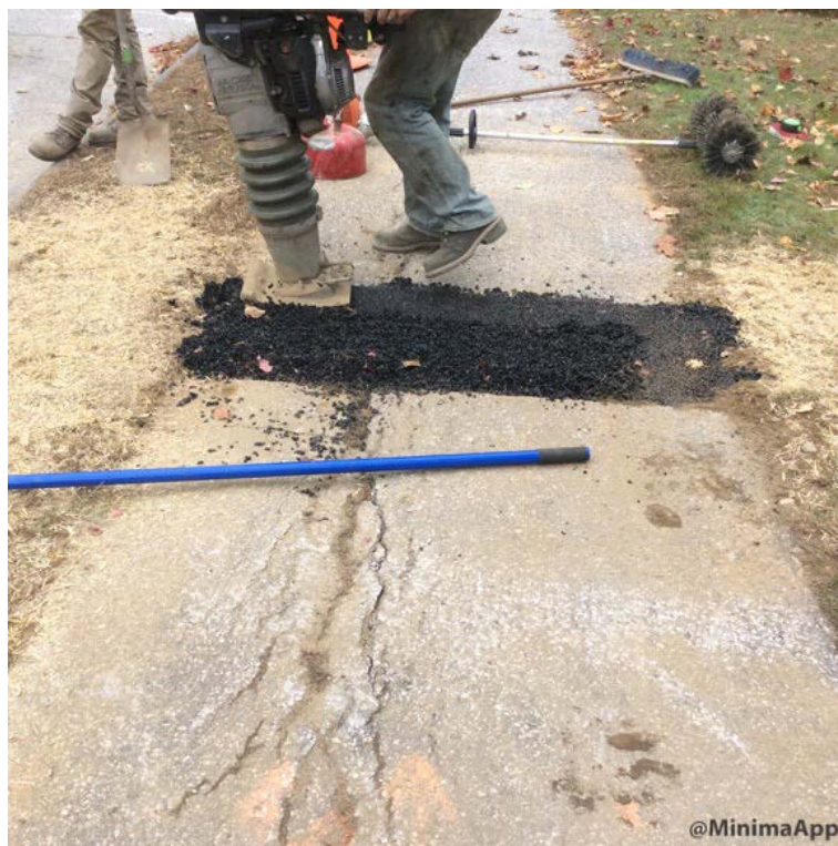
Compacting cold patch in sidewalk trench on Main Street
