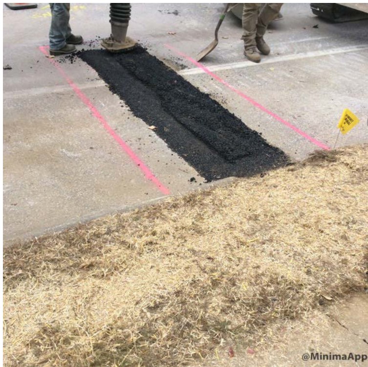
Compacting cold patch in roadway shoulder on Main Street
