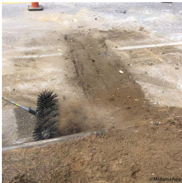
Compacted backfill in shoulder trench on Main Street.
