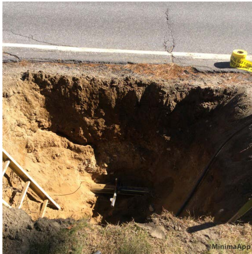
Trench excavated outside of roadway to access gas main for service connection.
